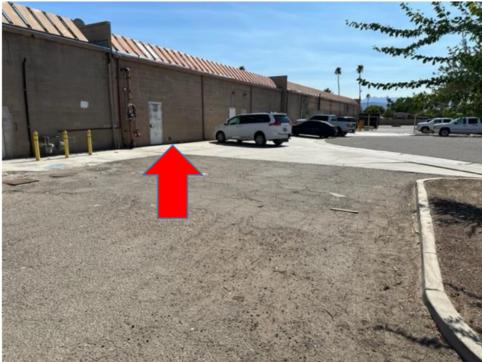
Rear View of Tenant Space
