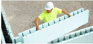
INSULATED CONCRETE FORM (ICF BLOCKS)
