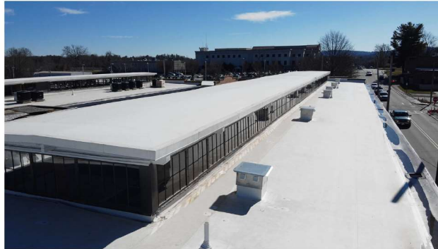
EXAMPLE OF THERMOPLASTIC POLYOLEFIN (TPO) ROOF CLASS "A" FIRE RATED
