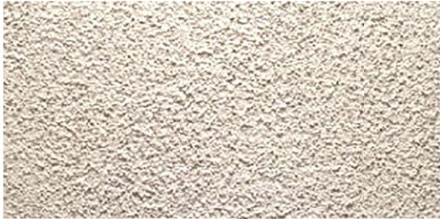
EXAMPLE OF TEXTURE OF A TRADITIONAL SAND FINISH STUCCO
