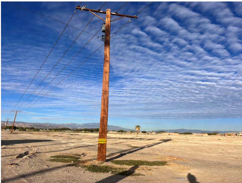
24. Pole-mounted transformer located along the southern property boundary – view facing northwest.
