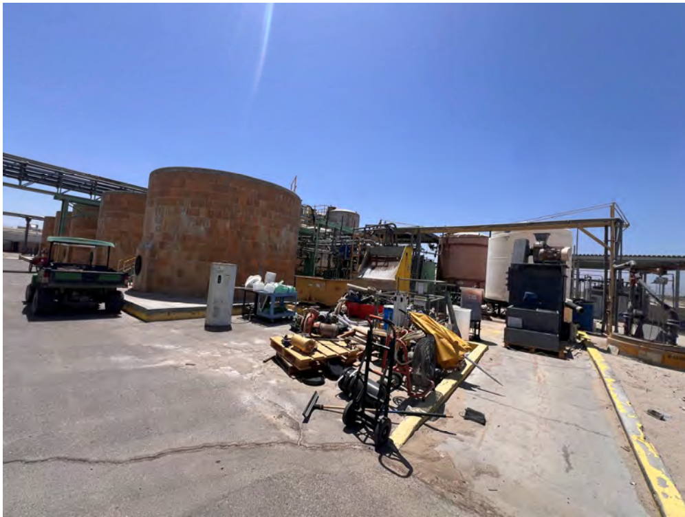
13. Typical 30,000-gallon slurry aboveground storage tanks (AST) shown to the left and water discharge system to the right.
