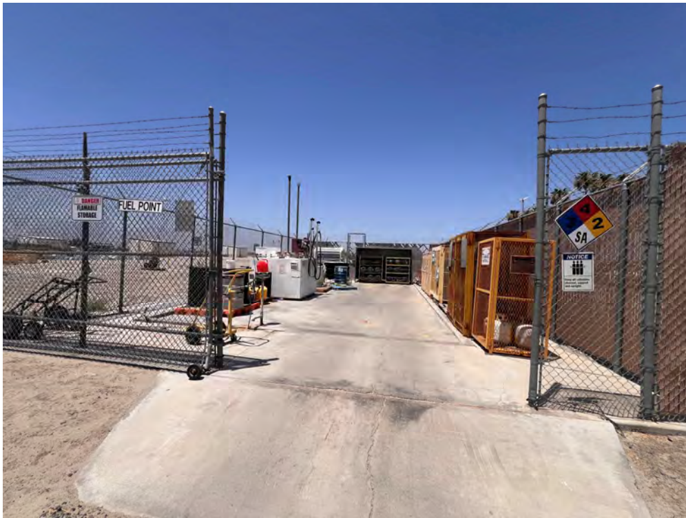
19. View of the fuel point, which contained a 1,500-gallon diesel AST, a 1,500-gallon gasoline AST, propane tanks, nitrogen tanks, and waste fuel/oil drums.
