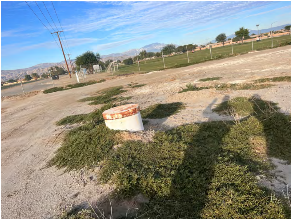
22. Concrete manhole reportedly used for sampling agricultural runoff – view facing west.
