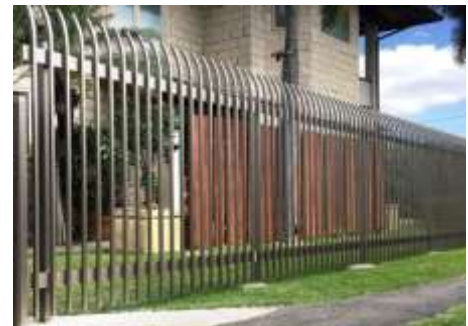
Figure 2 Wrought Iron Fencing Example
