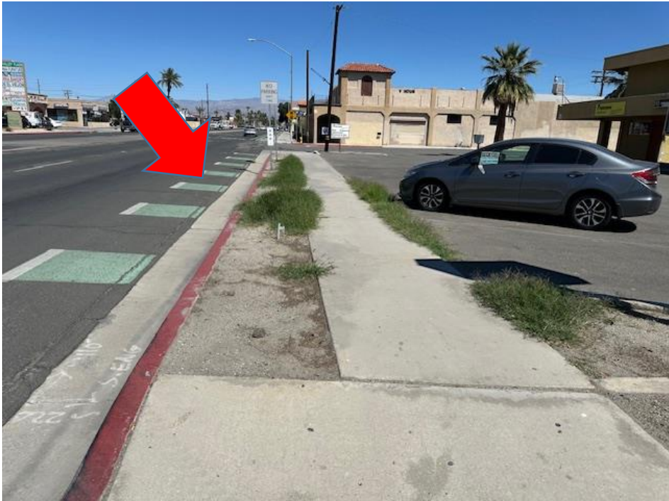
Landscaping – Cesar Chavez Street Frontage
