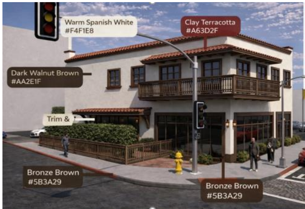
Figure 6 - Office/Clubhouse West Elevation (visible from Harrison Street)
