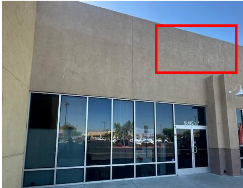
Exterior Surface Condition
