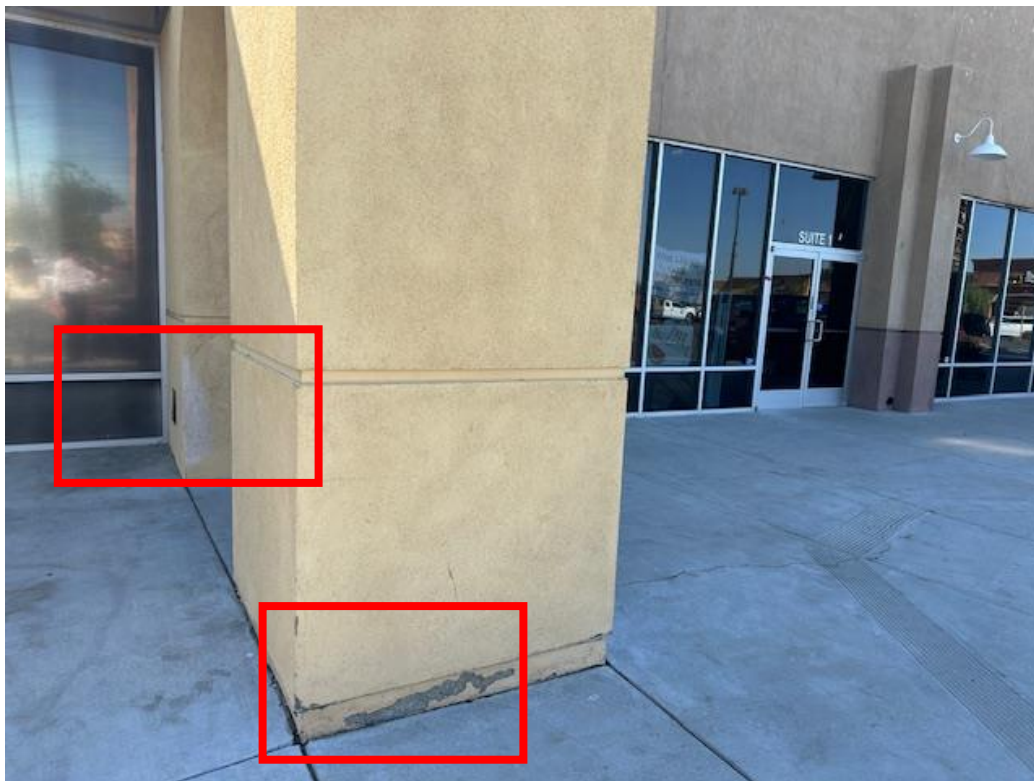
Exterior Surface Condition
