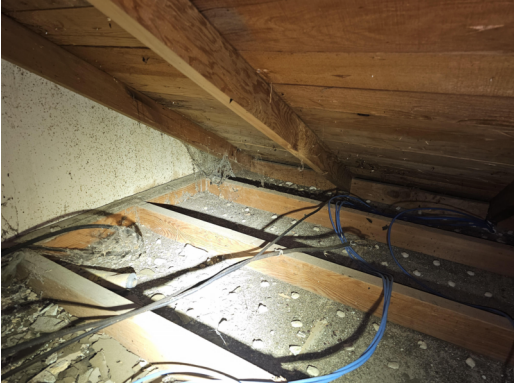
No shear transfer between the roof/ceiling diaphragm and shear walls
