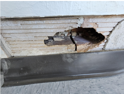
No reinforcement in clay/masonry walls
