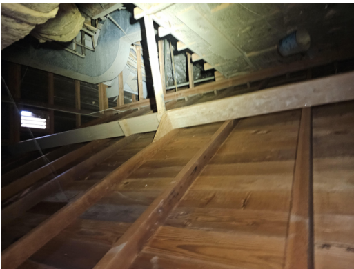
No positive connections of the post supporting the roof beams
