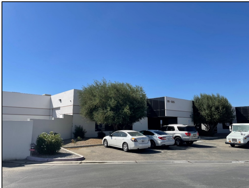
Industrial Building to the East of subject site
