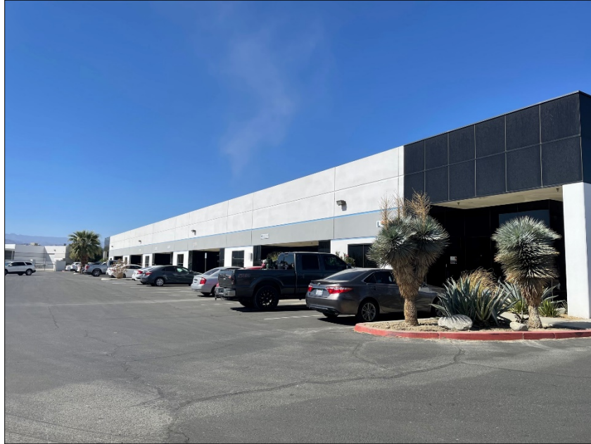
View of Existing Building and Parking lot looking West
