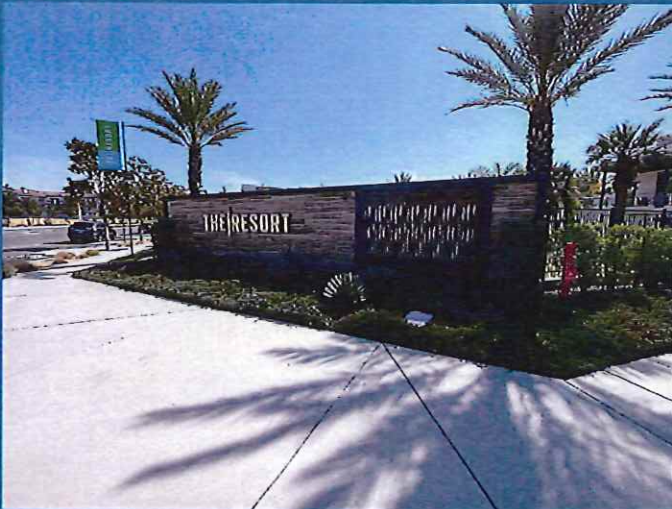
Before Site Improvement
