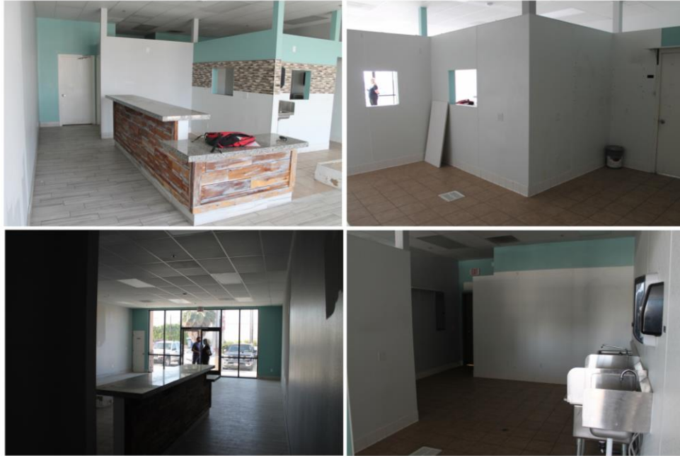
Current condition of the unit
