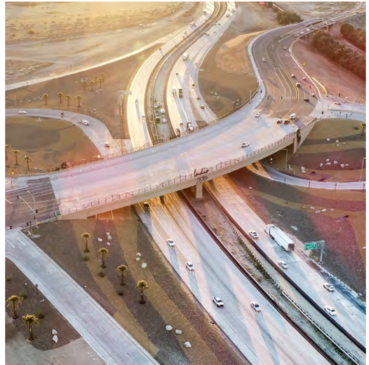
Figure 2. I-10/Jefferson Street Interchange
