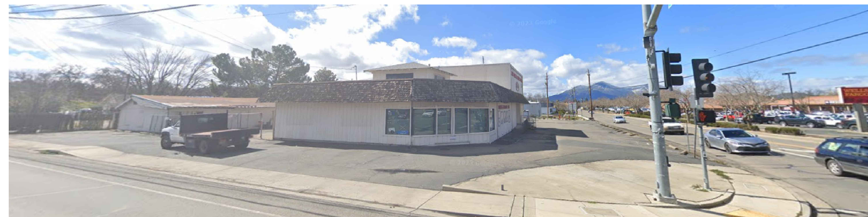
CORNER VIEW @ OLD HIWAY 53 AND OLYMPIC DR.
