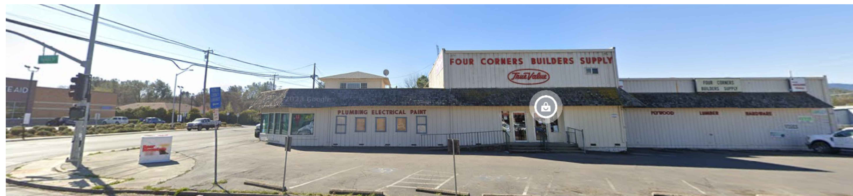
CORNER VIEW @ OLYMPIC DR. AND OLD HIWAY 53
