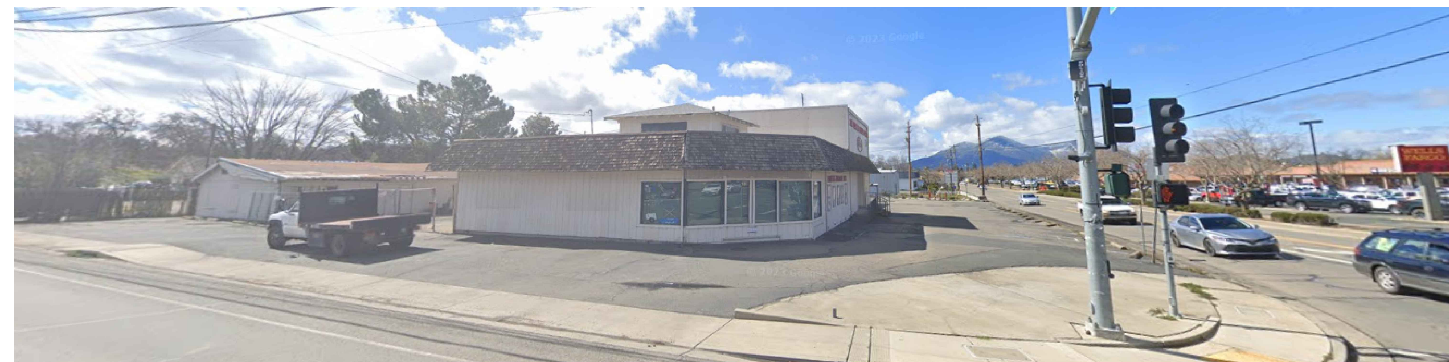
CORNER VIEW @ OLD HIWAY 53 AND OLYMPIC DR.
