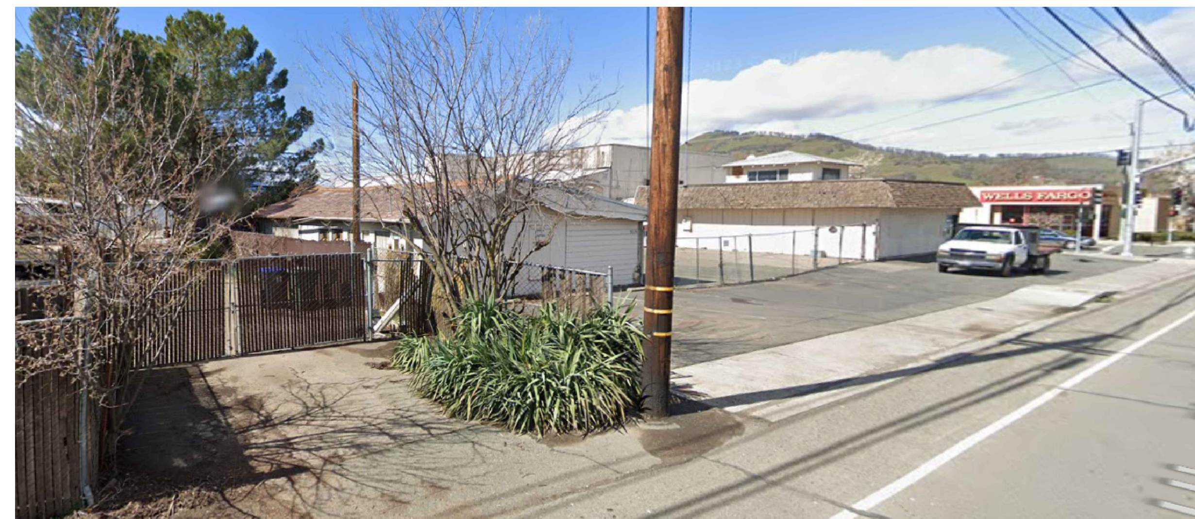
EAST SIDE ALONG OLD HIWAY 53
