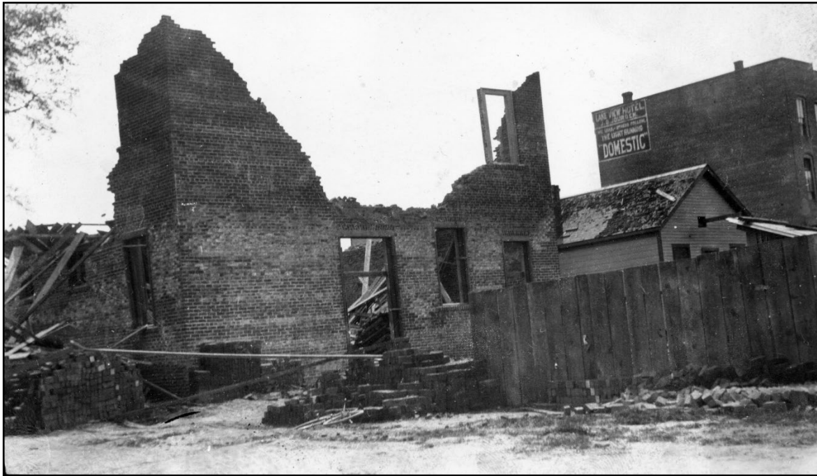
Figure 7: Possible 1906 Earthquake Damage (Lakeport)
