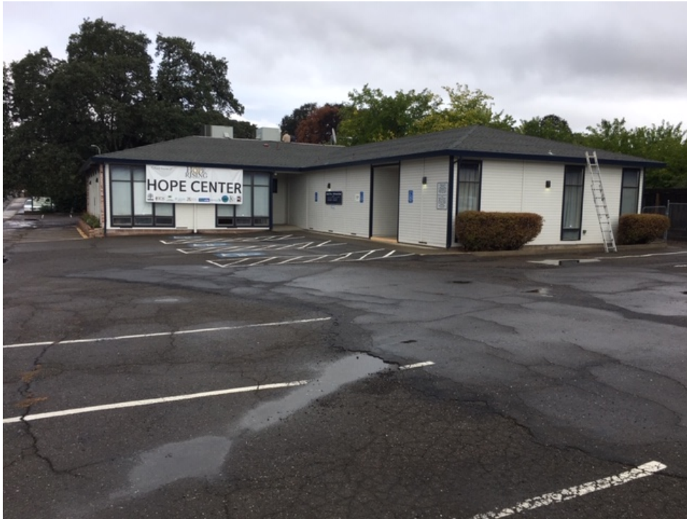
Photo No. 1: Northeasterly view project building and site from the intersection of Emerson and Olympic
