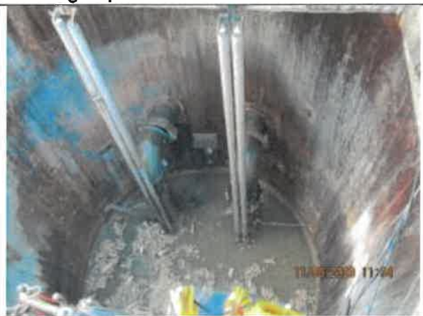
Photo 12: A photo of the south wet well at Pump Station No. 2 showing minor debris, FOG, and staining on the walls. The disconnected pipe in the photo is currently under repairs.
