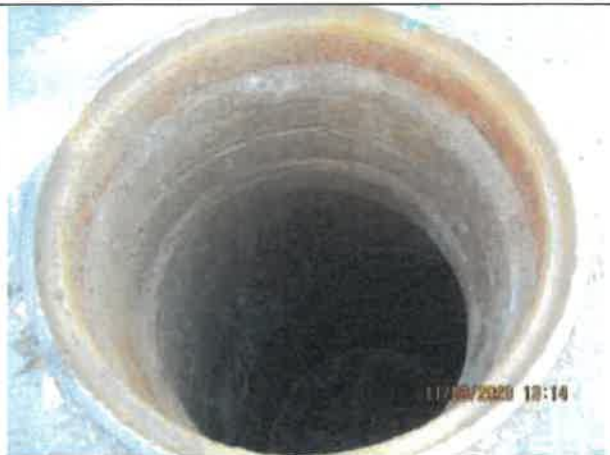
Photo 22: A photo on the manhole located at the intersection of Bay Street and Lakeview Way with corrosion around the rim and staining in the barrel.
