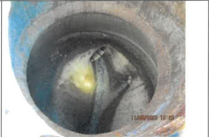
Photo 24: A photo on the manhole located in front of 6825 Meadowbrook Drive low flow and FOG on the sides of the manhole channel.
