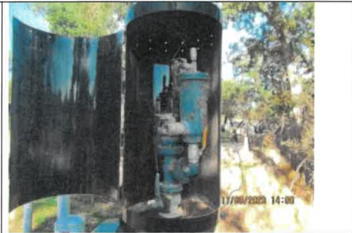
Photo 31: A photo of the ARV located at the aerial crossing with cobwebs around the ARV.
