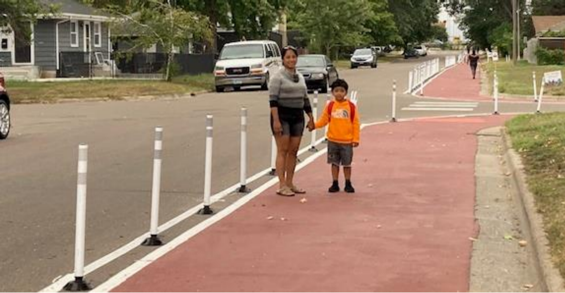
Example of an 11' shared use path with vertical barriers
