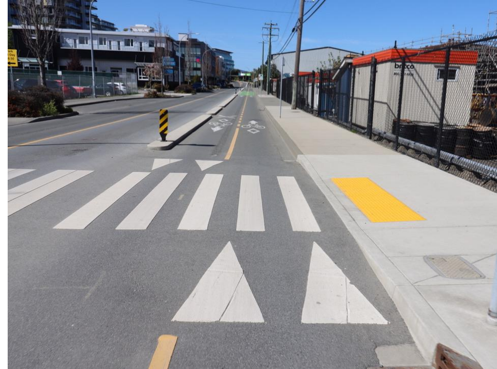
Raised crossing for a bike facility (Victoria, B.C.)
