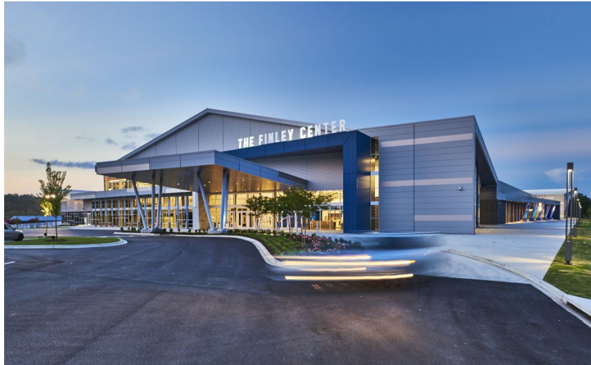
Figure 7: Burns Valley Sports Complex Park Project 15,000 square foot Community Center Building Concept and Example of Buildings
