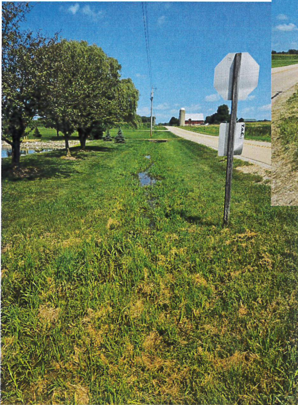
▲ 7 – West Ditch of Island Road Looking North
