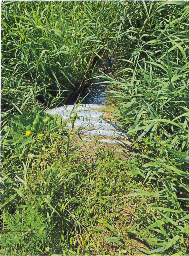
▲ 1 - Culvert on South Side of Winnegamie Drive
