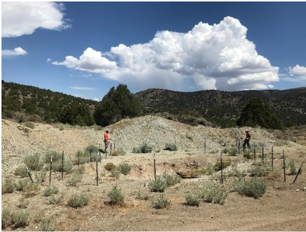
Photo 3 - AML Interns building a fence, Washoe County, Nev.
