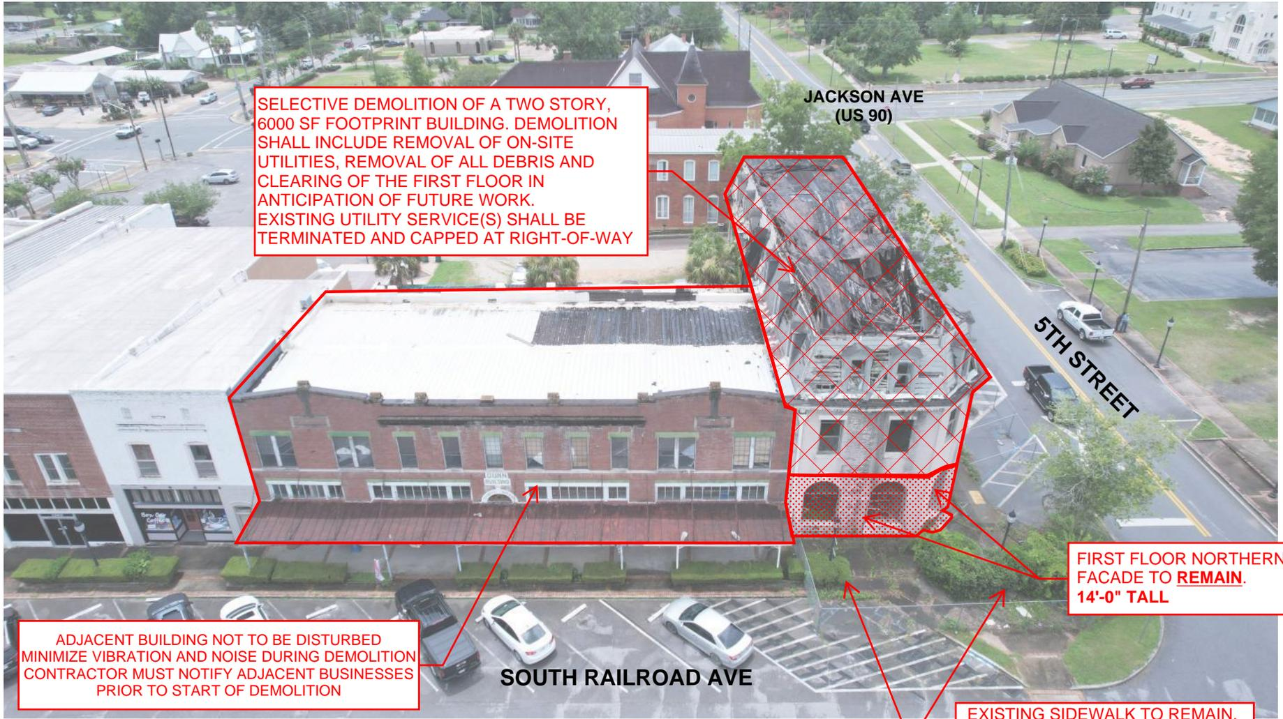
SELECTIVE DEMOLITION OF A TWO STORY, 6000 SF FOOTPRINT BUILDING. DEMOLITION SHALL INCLUDE REMOVAL OF ON-SITE UTILITIES, REMOVAL OF ALL DEBRIS AND CLEARING OF THE FIRST FLOOR IN ANTICIPATION OF FUTURE WORK. EXISTING UTILITY SERVICE(S) SHALL BE TERMINATED AND CAPPED AT RIGHT-OF-WAY
