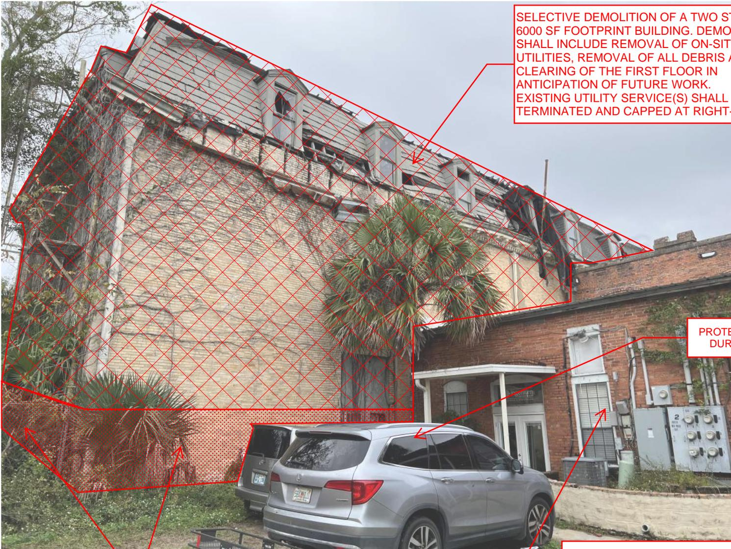
SELECTIVE DEMOLITION OF A TWO STORY, 6000 SF FOOTPRINT BUILDING. DEMOLITION SHALL INCLUDE REMOVAL OF ON-SITE UTILITIES, REMOVAL OF ALL DEBRIS AND CLEARING OF THE FIRST FLOOR IN ANTICIPATION OF FUTURE WORK. EXISTING UTILITY SERVICE(S) SHALL BE TERMINATED AND CAPPED AT RIGHT-OF-WAY
