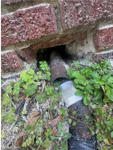
Figure 12 – Disconnected and/or Abandoned Pipe
