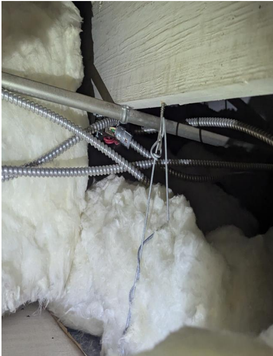
Figure 4: Exposed Wires from MC Type Sheathing
