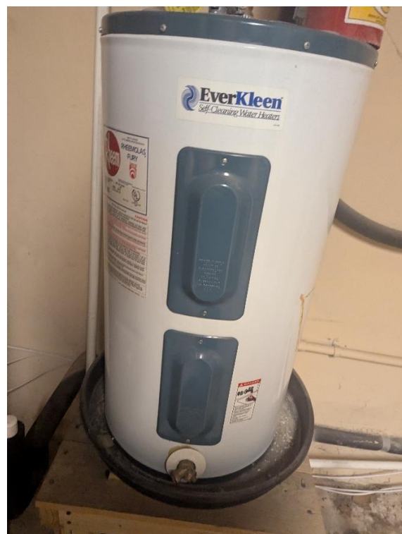
Figure 11 – Electric Tank Water Heater
