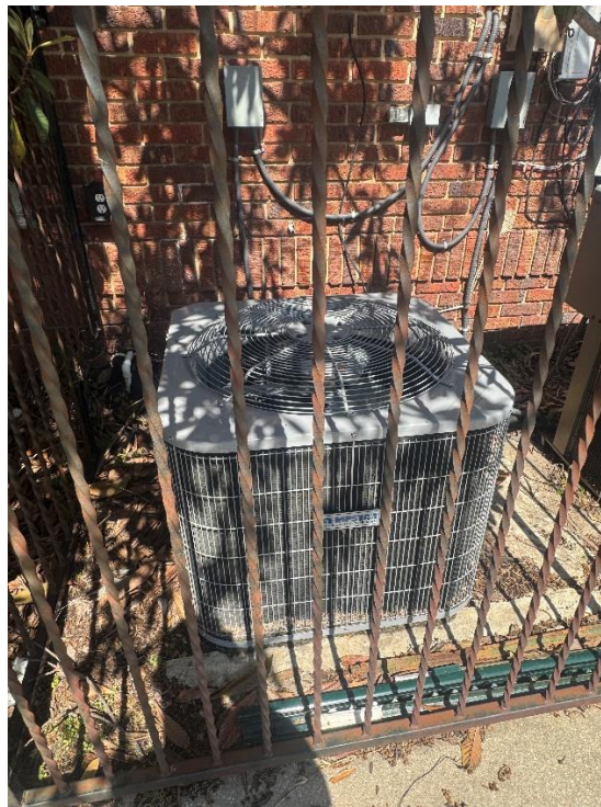
Figure 4 - Heat Pump Unit (HPU-2)
