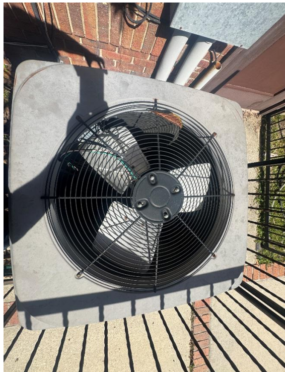
Figure 2 – Heat Pump Unit (HPU-1)
