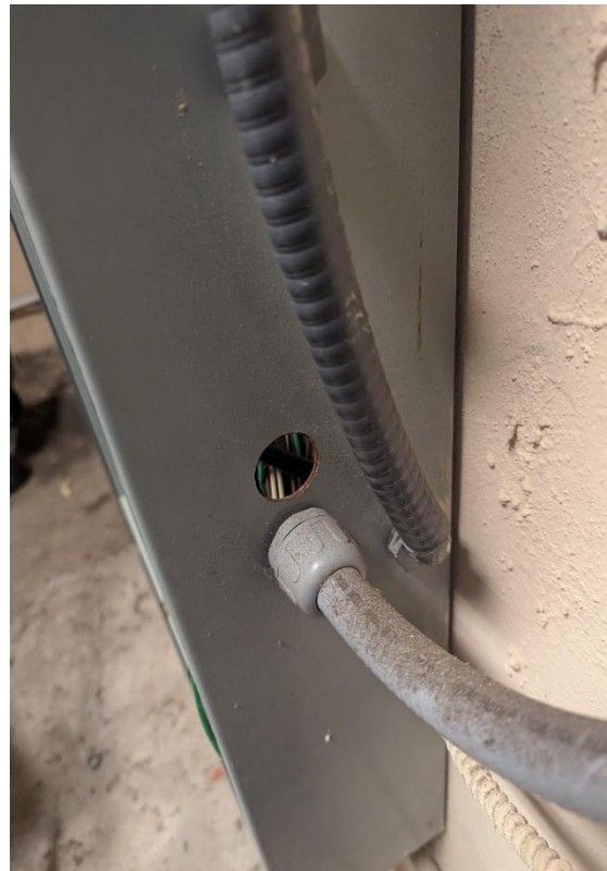
Figure 7: Exposed Electrical Gap
