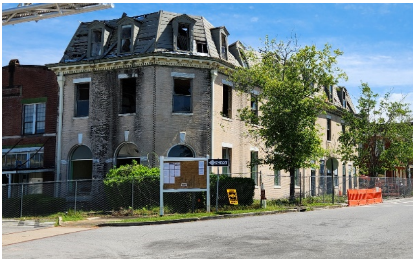
Photo 17. The remnants of a former bank building at the southeast corner of South Railroad Avenue and 5 th Street is scheduled for removal this year.
