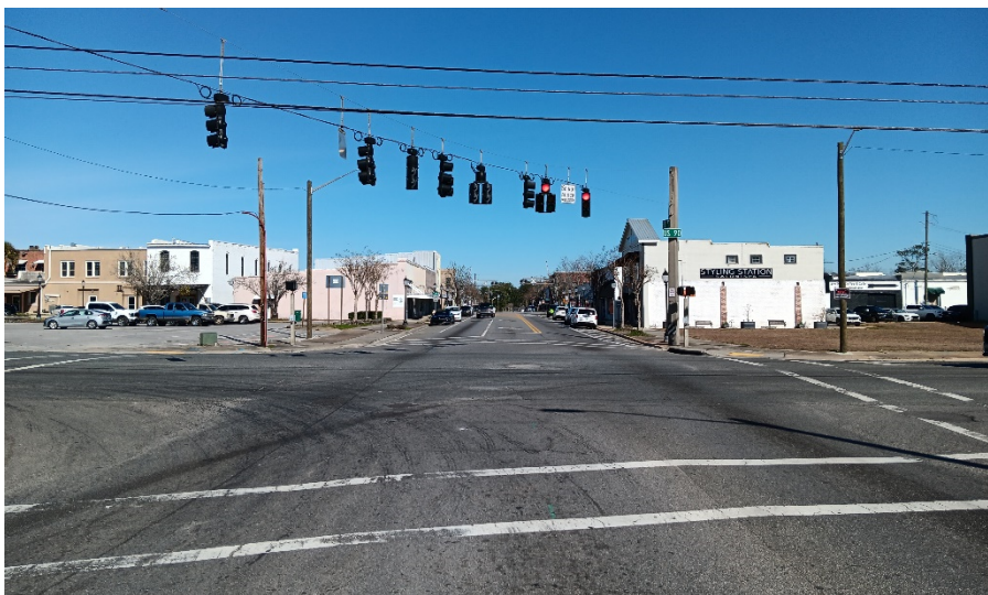
Photo 24. Inadequate crosswalk definition at the intersection of Jackson Avenue (US Highway 90) and Main Street (SR 77) represents a safety hazard for pedestrians. Also, large parking areas without plantings contribute to the lack of identity in this area.
