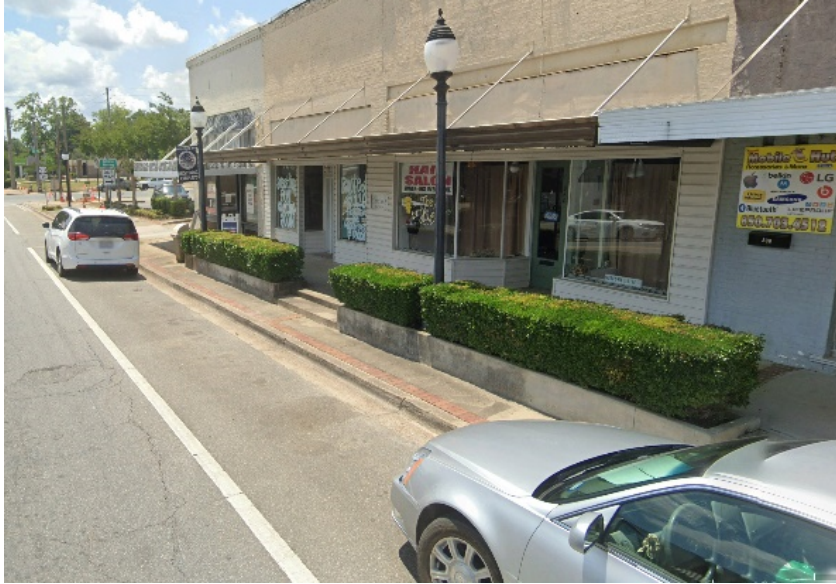
Photo 15. Another example of inappropriate modifications to historic buildings, including boarding over clerestory windows, covering of brick with stucco or plywood, and addition of various awning materials.
