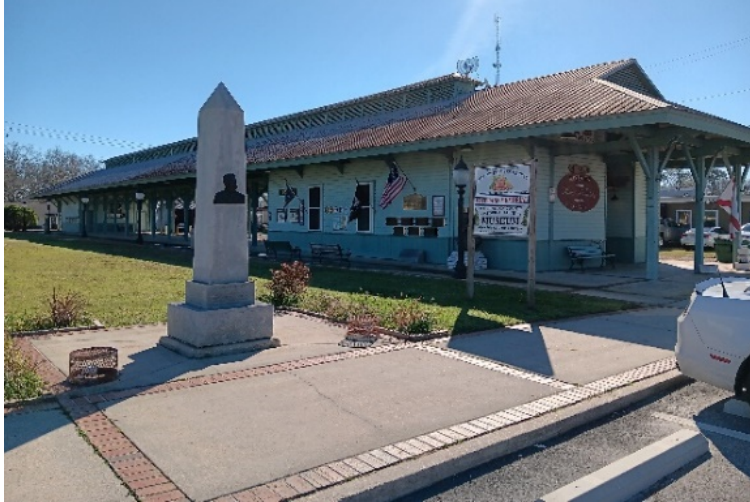
Photo 9. Washington County Historical Society Museum and Chipley Farmers Market, housed in re-creation of depot building.
