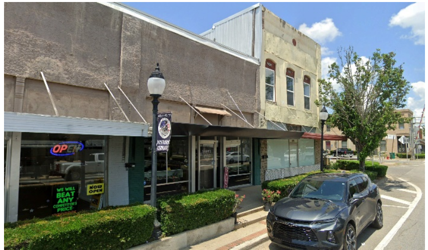
Photo 16. Inappropriate cladding of historic storefront, using unpainted boards.
