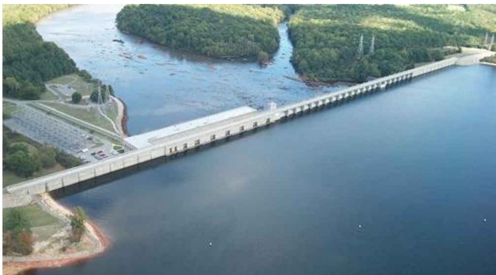
John H. Kerr Dam and Reservoir. Photo credit: US Army Corps of Engineers.
