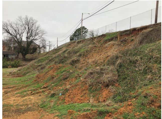
(Left) A small mudslide occurred on US 58 between South Boston and Danville due to the effects of Tropical Storm Michael in October of 2018. Photo Credit: Ginger New.
