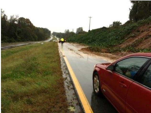
(Left) A small mudslide occurred on US 58 between South Boston and Danville due to the effects of Tropical Storm Michael in October of 2018. Photo Credit: Ginger New.
