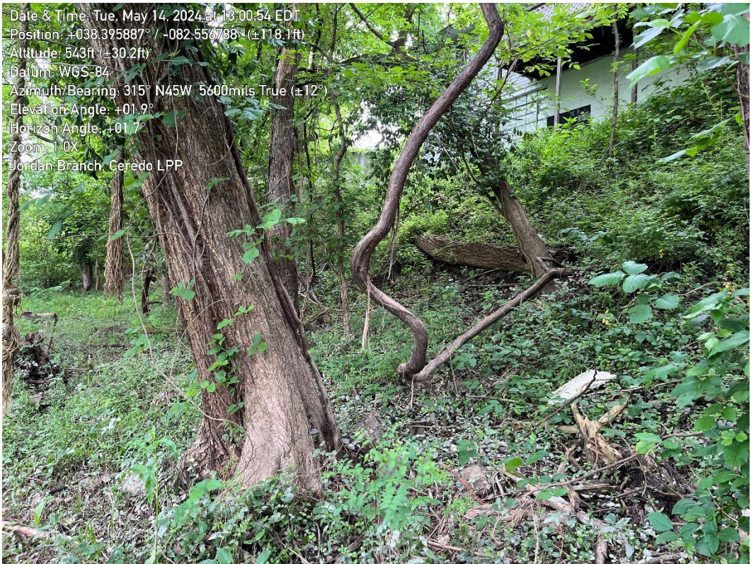
Figure 5. Trees within the slope are misaligned.
