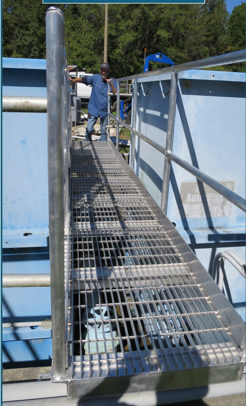
New Catwalk on Filters
