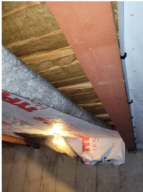
Bottom of Steel Beam
