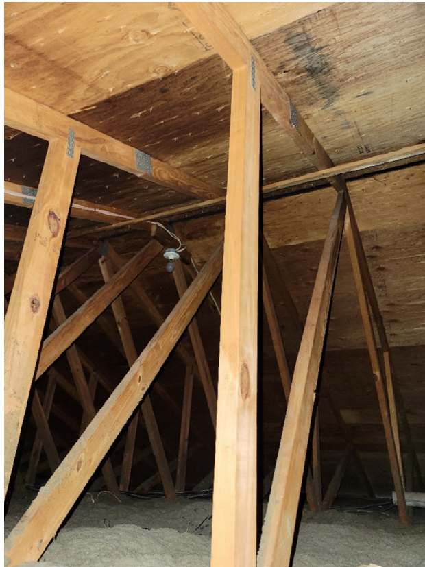
Wood Rood Trusses
