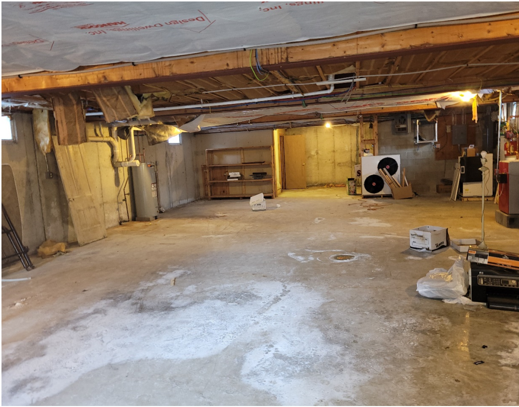
View of Basement
