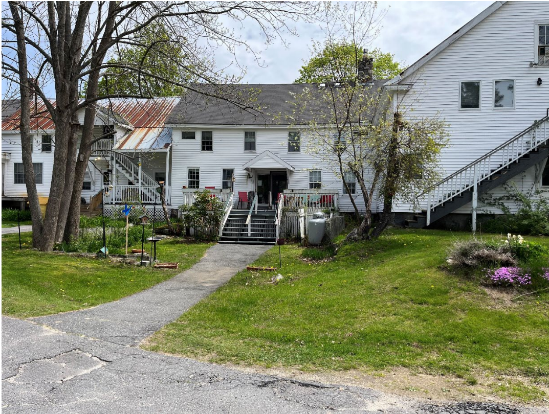
PHOTO 1 – LOOKING AT REAR OF EXISTING FACILITY.
