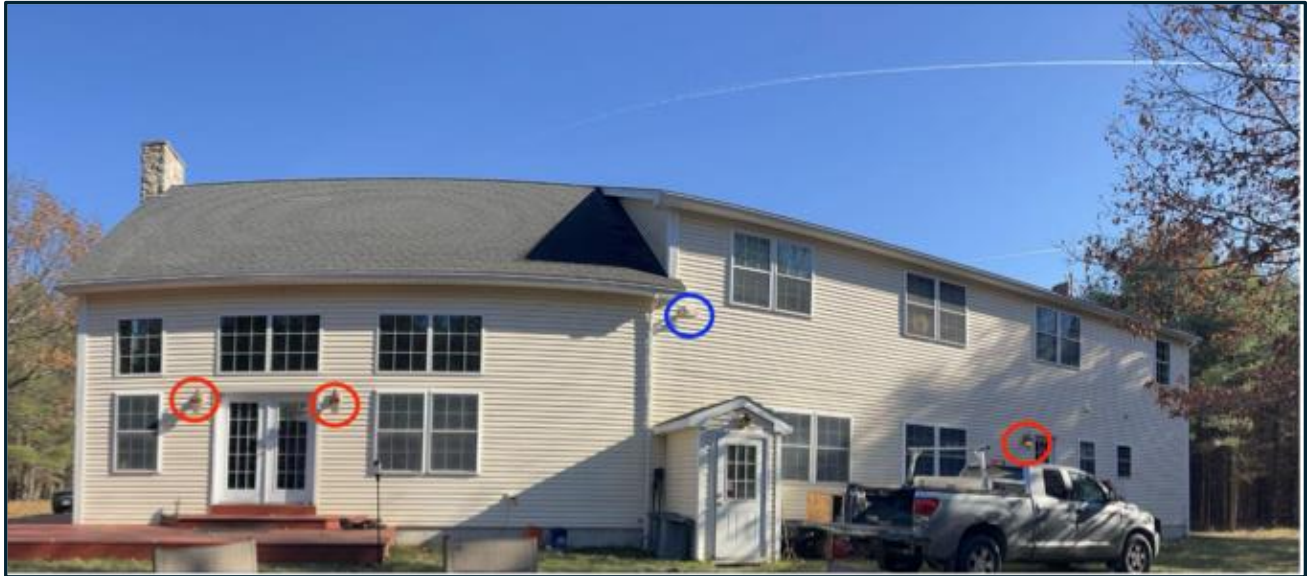
Back: 3 Lantern-style scones and 1 floodlight above the back door.
