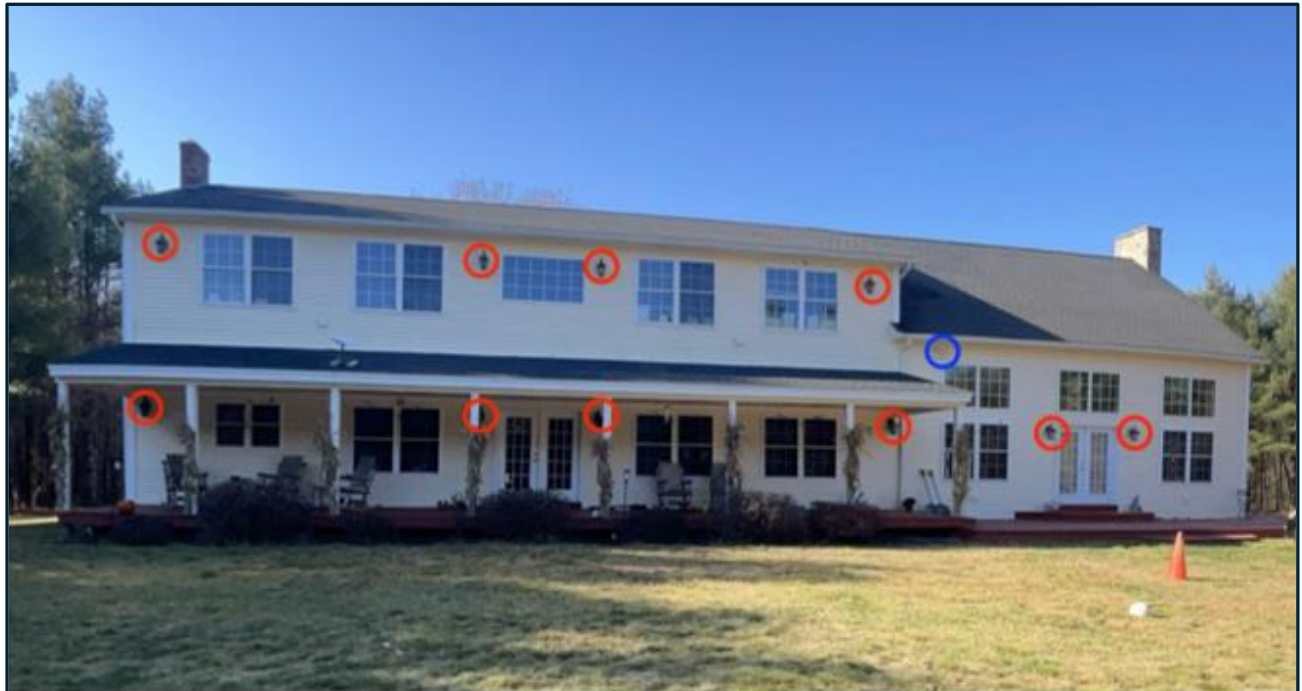
Front: 10 lantern-style scones and 1 floodlight on the porch.
