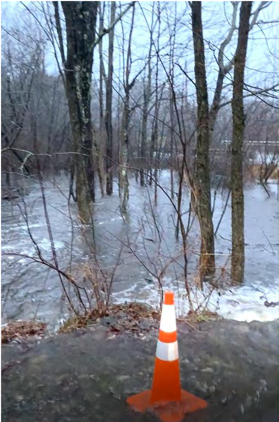
High Water – Looking at Culvert Inlet from Davis Brook Road (taken December 2023)
