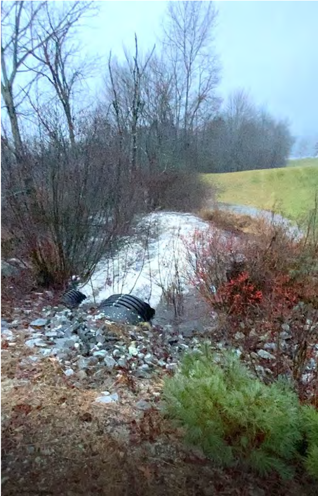
High Water – Looking at Culvert Outlet from Edwards Road (taken December 2023)
