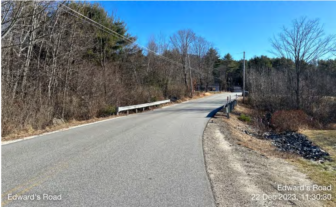
Edwards Road where it crosses Edwards Brook.
