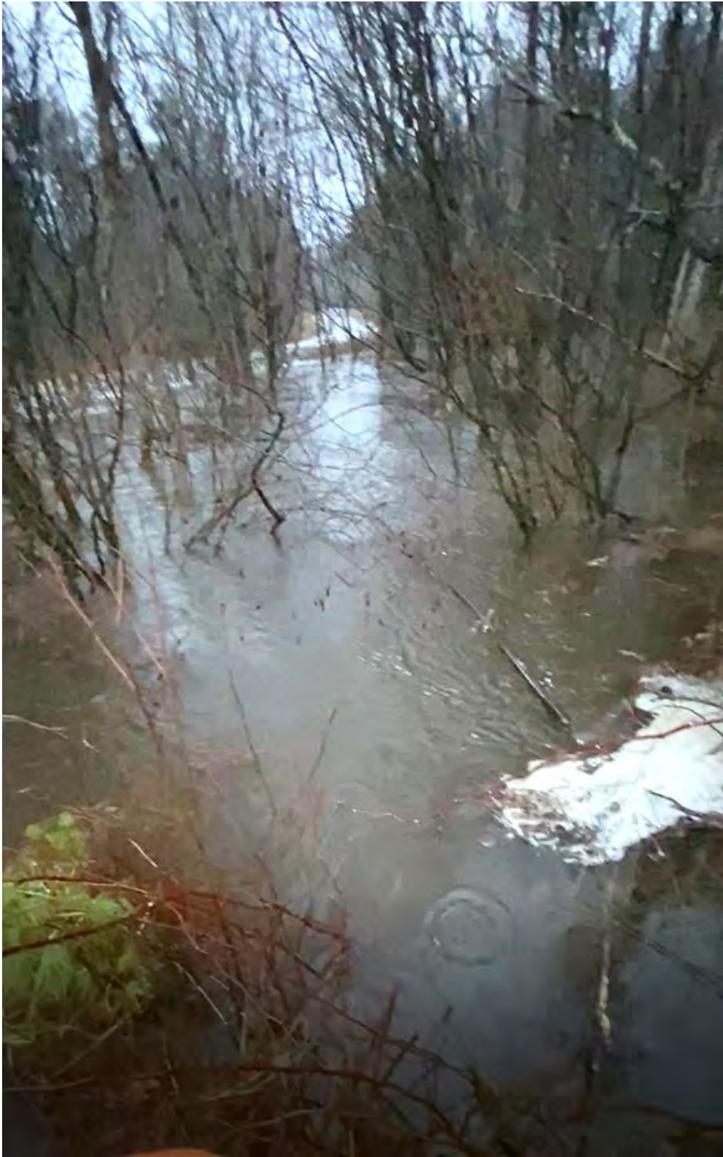
High Water – Looking at Culvert Inlet from Edwards Road (taken December 2023)
