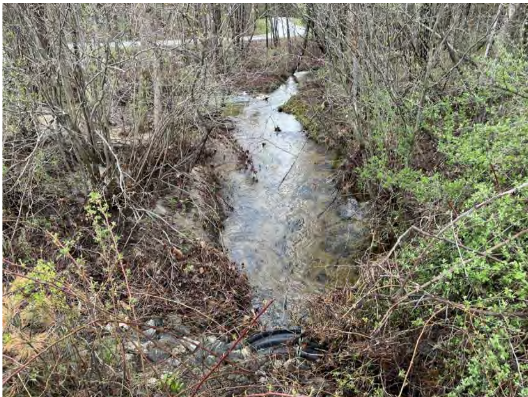
Inlet – Looking Upstream (taken May 4, 2023)
