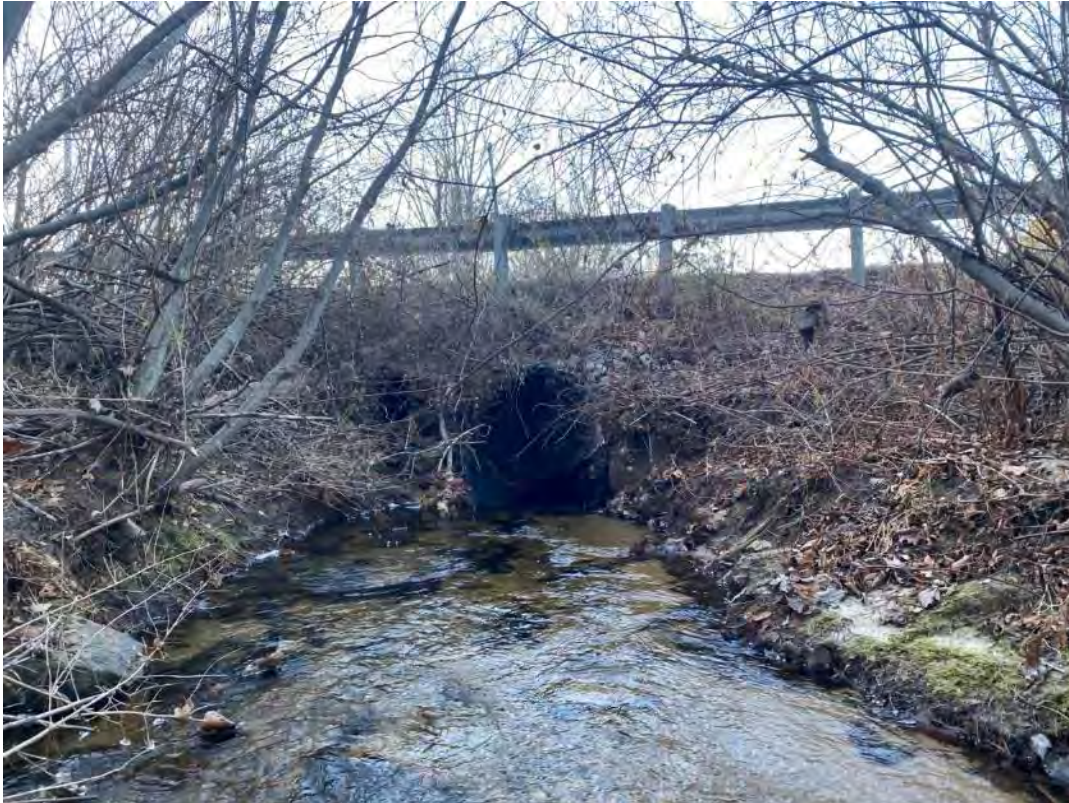
Inlet – 18" and 48" HDPE Culverts (taken May 4, 2023)
