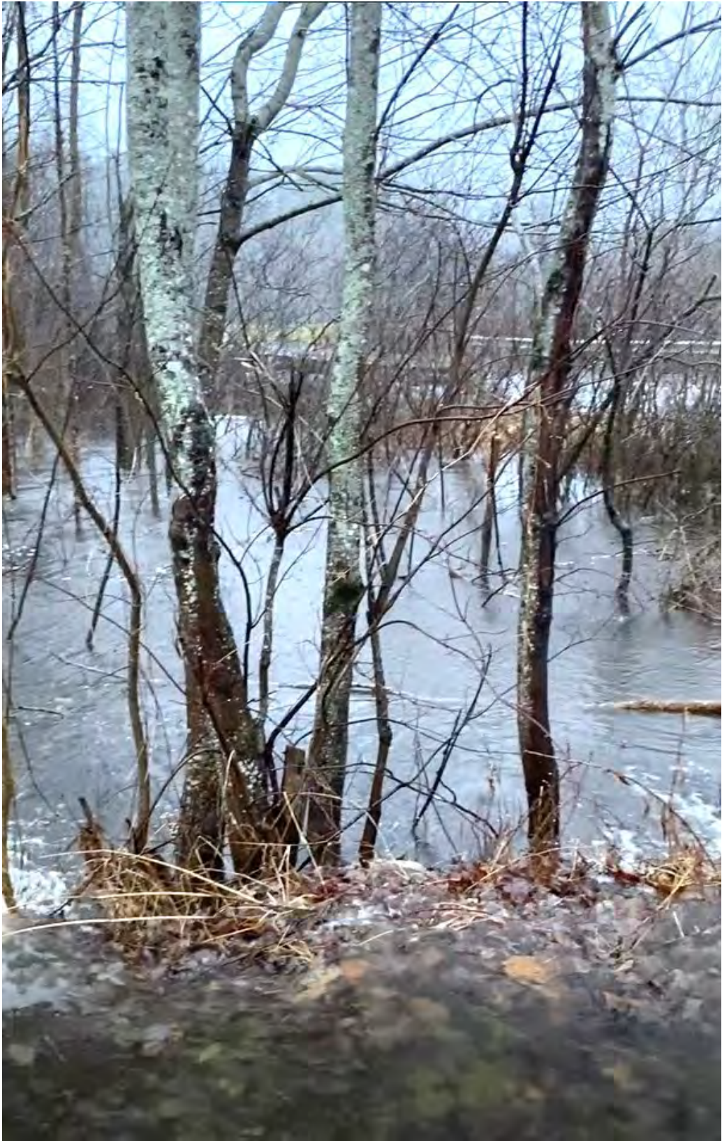
High Water – Looking at Culvert Inlet from Davis Brook Road (taken December 2023)
