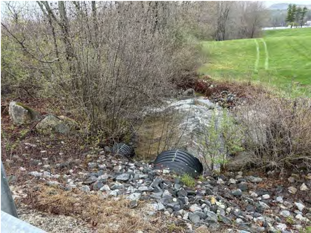
Outlet – Looking Downstream (taken May 4, 2023)
