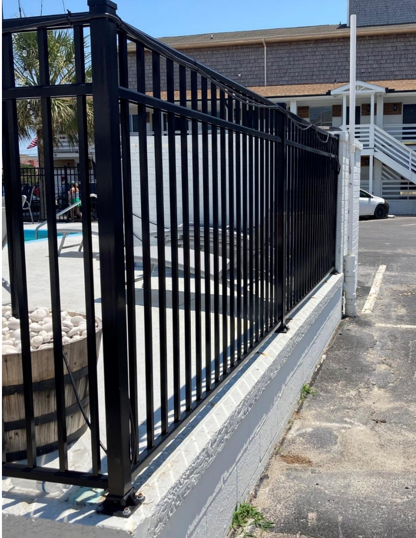
Current Fencing Compared to Brick Pump House
