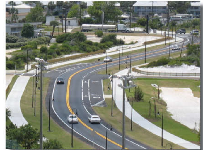
Commons Drive incorporates all multimodal components of roadway design.
