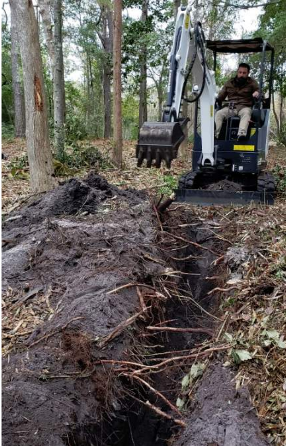
Figure 19. Excavating the trench adjacent to the southern site border.
