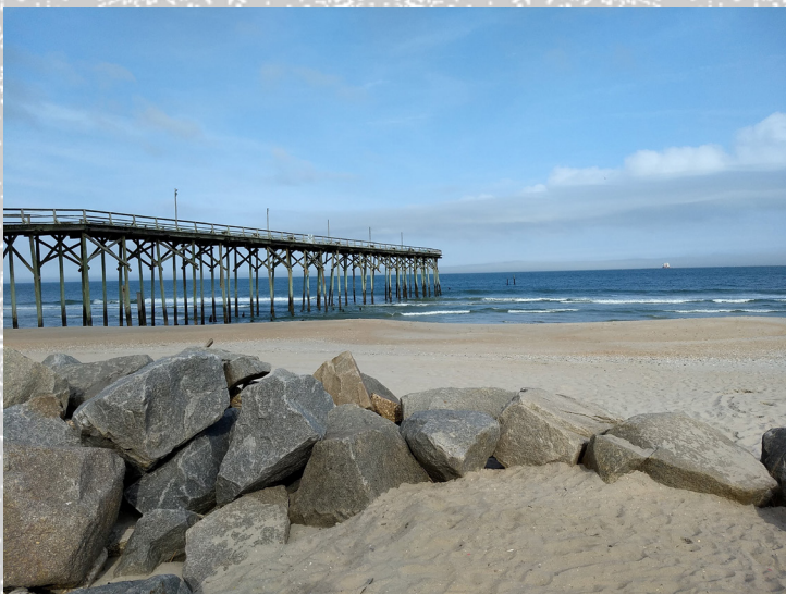
The pier on the North End.
