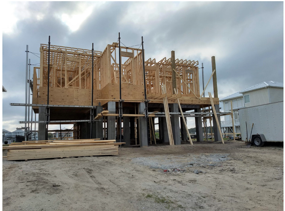
Although no building code regulations can completely protect against rising seas and increasingly damaging storms, significant elevation of new structures will help reduce vulnerability to stormwater flooding.
