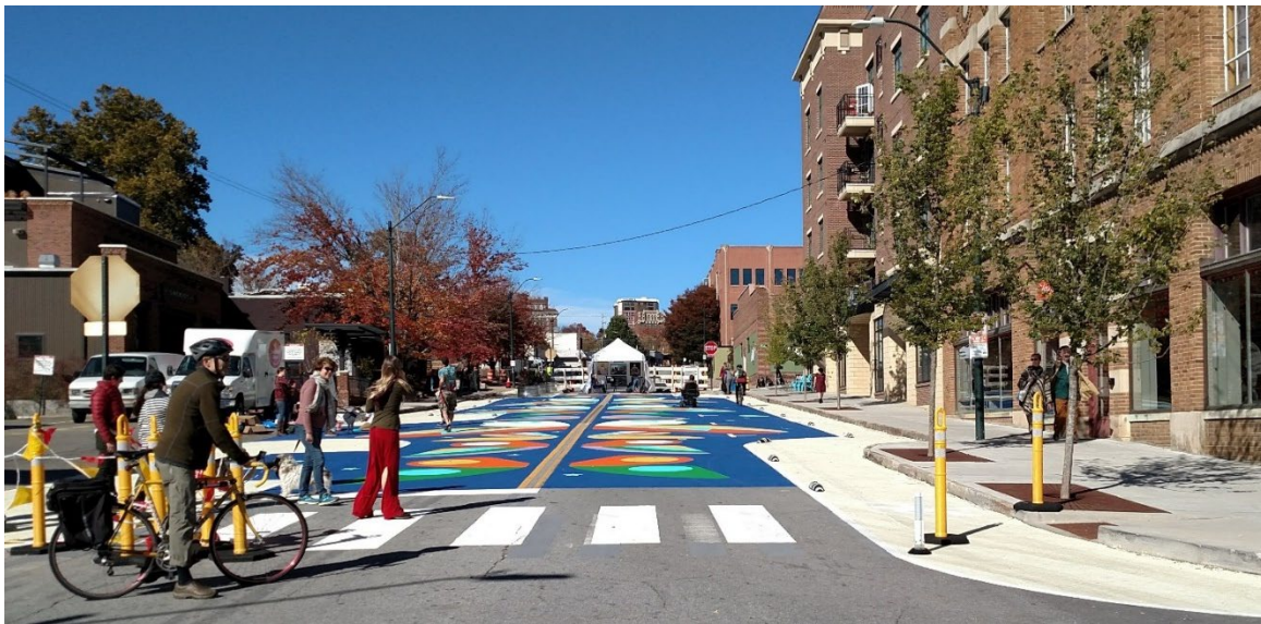
Temporary installation of a street mural and separated bike lanes (Asheville, NC)
