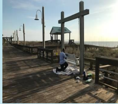
Staining and maintenance of Boardwalk And Marina docks prior to Summer
