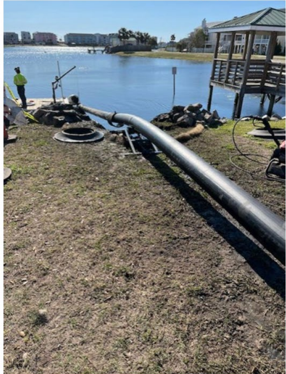
CB Lake is being treated for algae, duckweed, and parrotfeather; #3 lake pump pipe repaired
