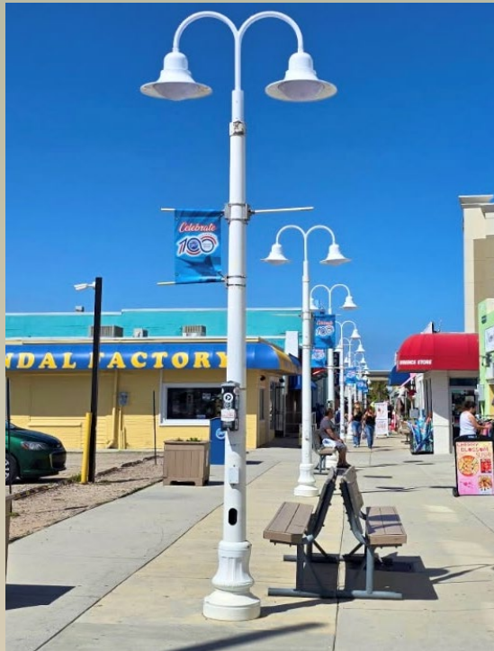
Replacement of all Town lamp lights and sunshades
