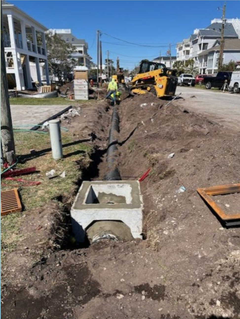
Updated stormwater added to the 1500 block of Mackerel Lane
