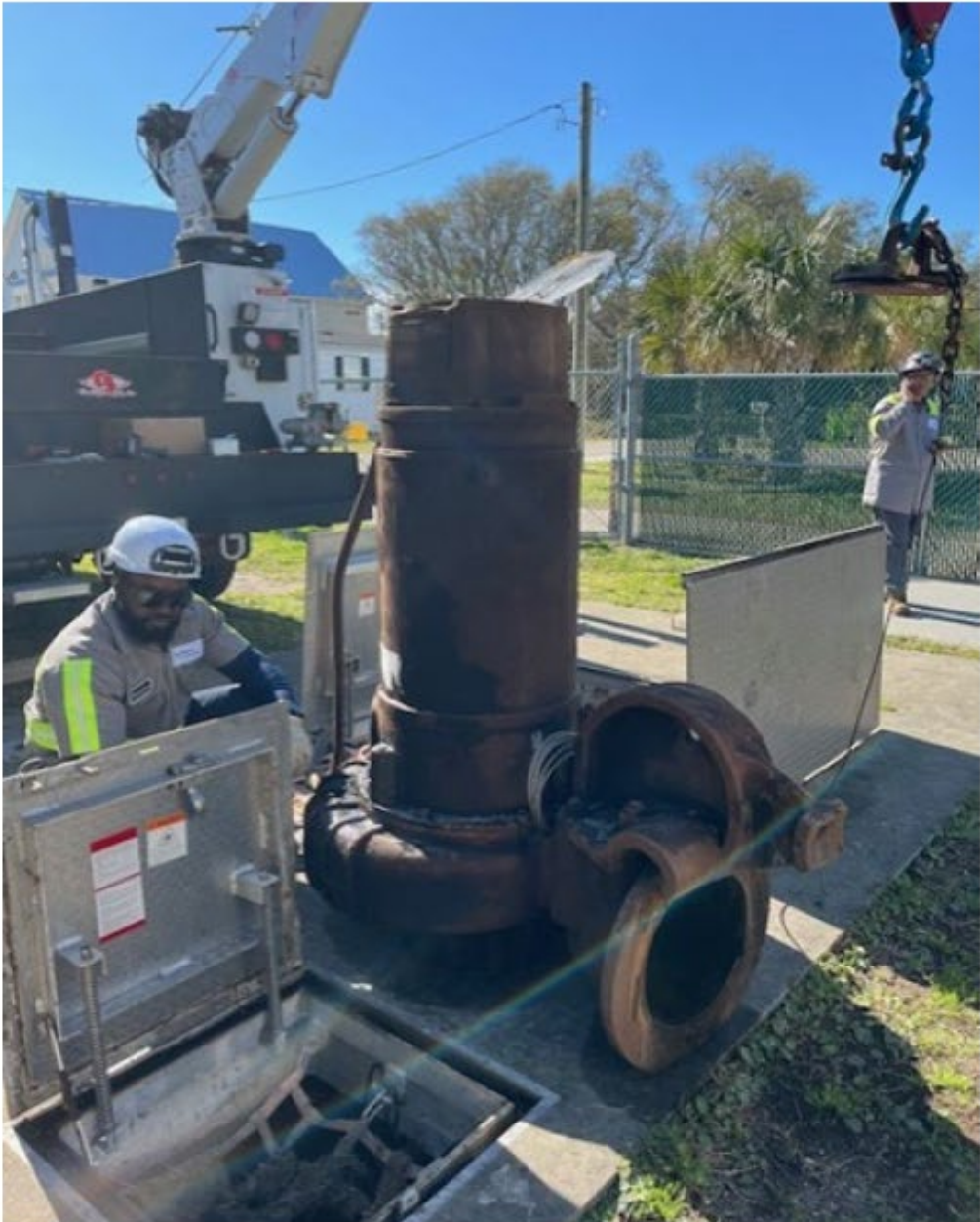
Texas Ave. pump was taken offsite for repairs
