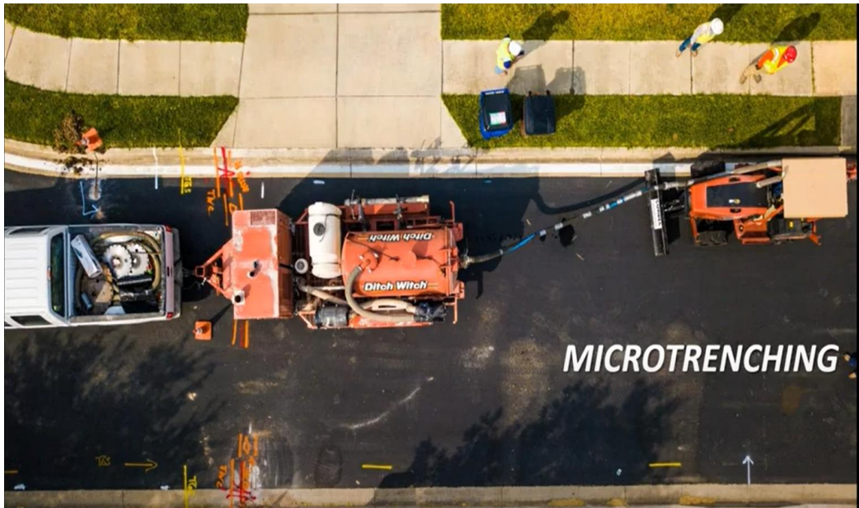
Figure 4: Trench in pavement (Microtrenching)
