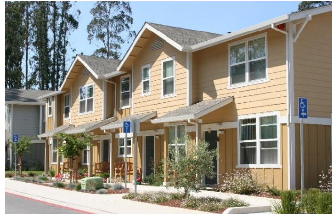
Parkhurst Terrace, Aptos, 68 units Family Housing
