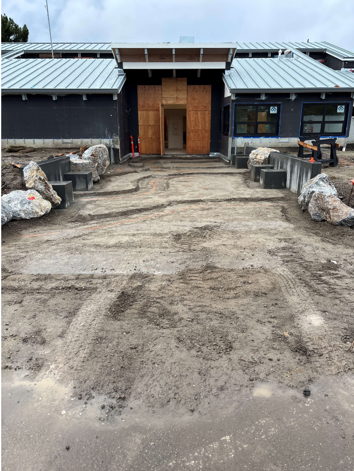
Front entry approach graded and compacted, with concrete seat walls and large boulders installed along the pedestrian pathway
