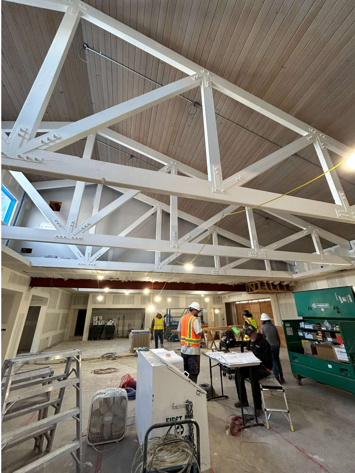
Exposed truss system fully painted
