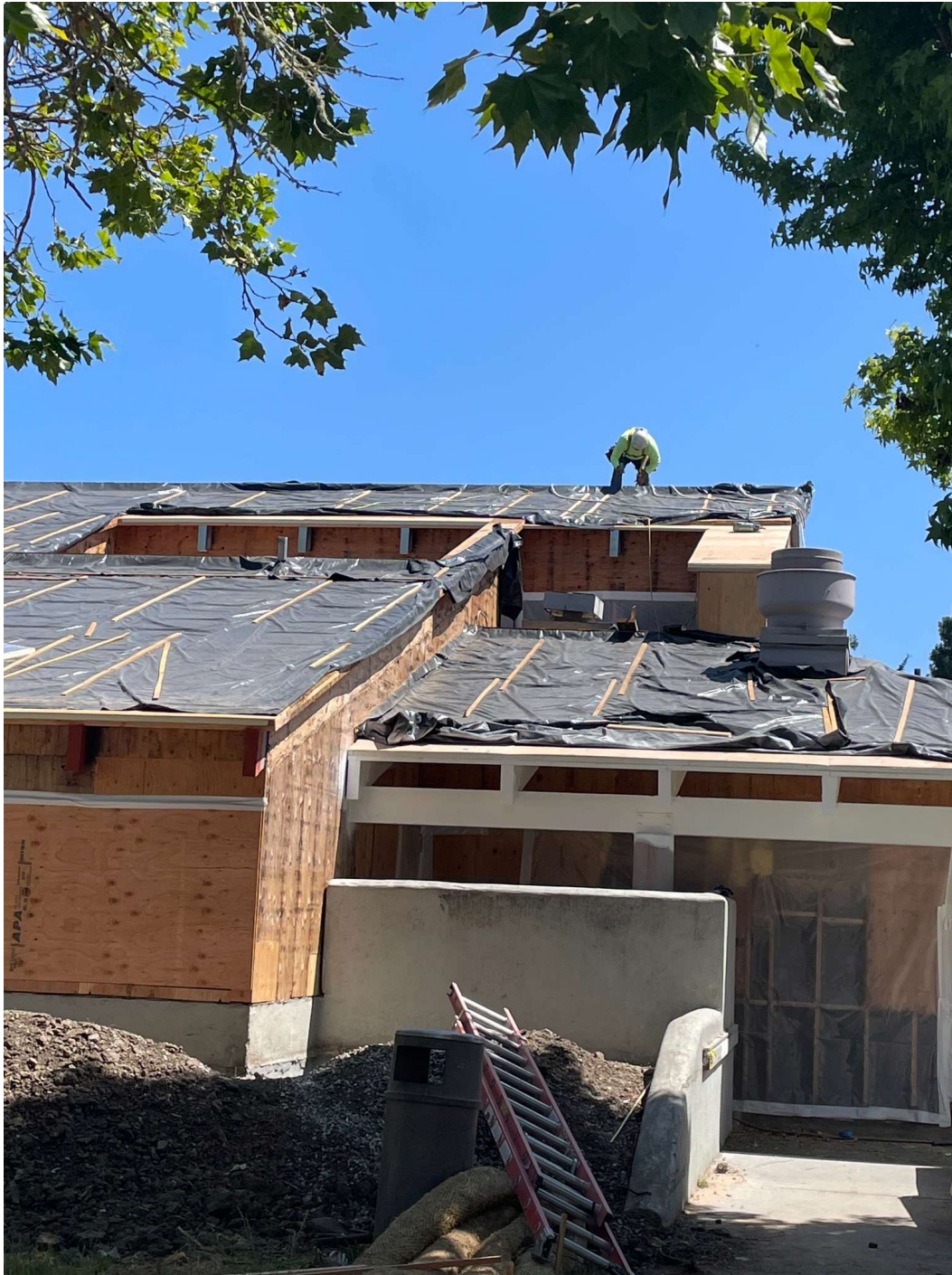
Crew working on roof structure, black sheathing in place for weather protection.
