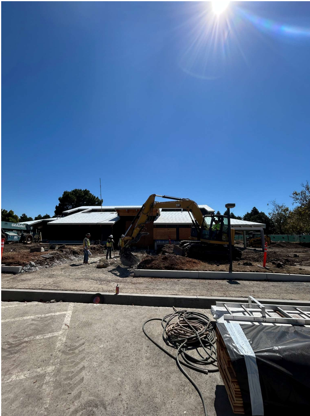
Heavy equipment and crews performing grading and concrete work at building entrance.
