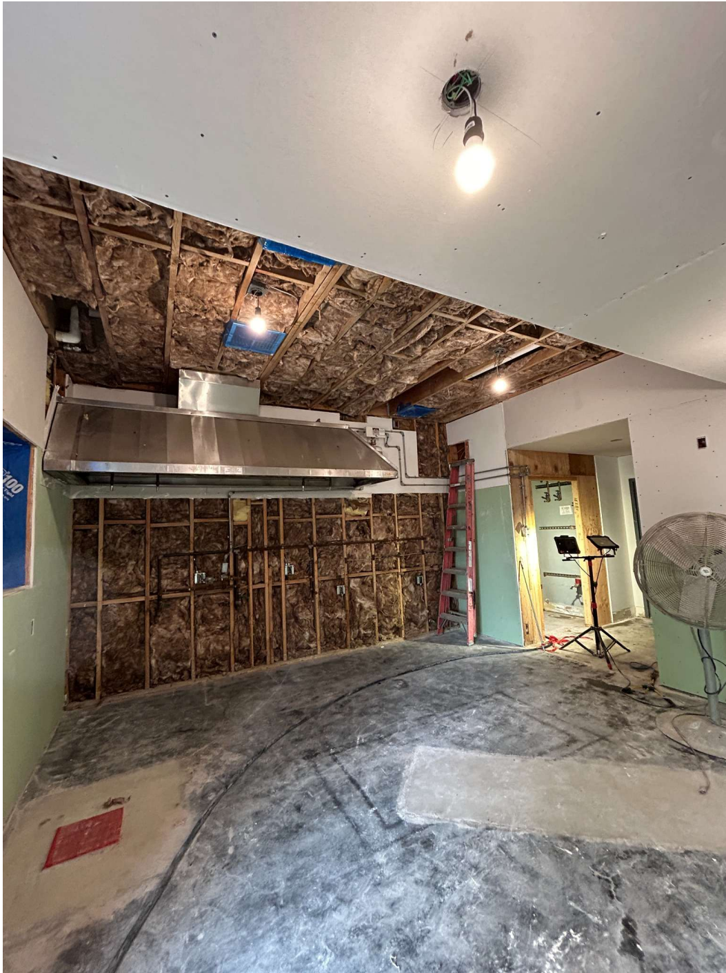
Exposed framing, insulation, and partial drywall installation with ceiling electrical rough-ins.
