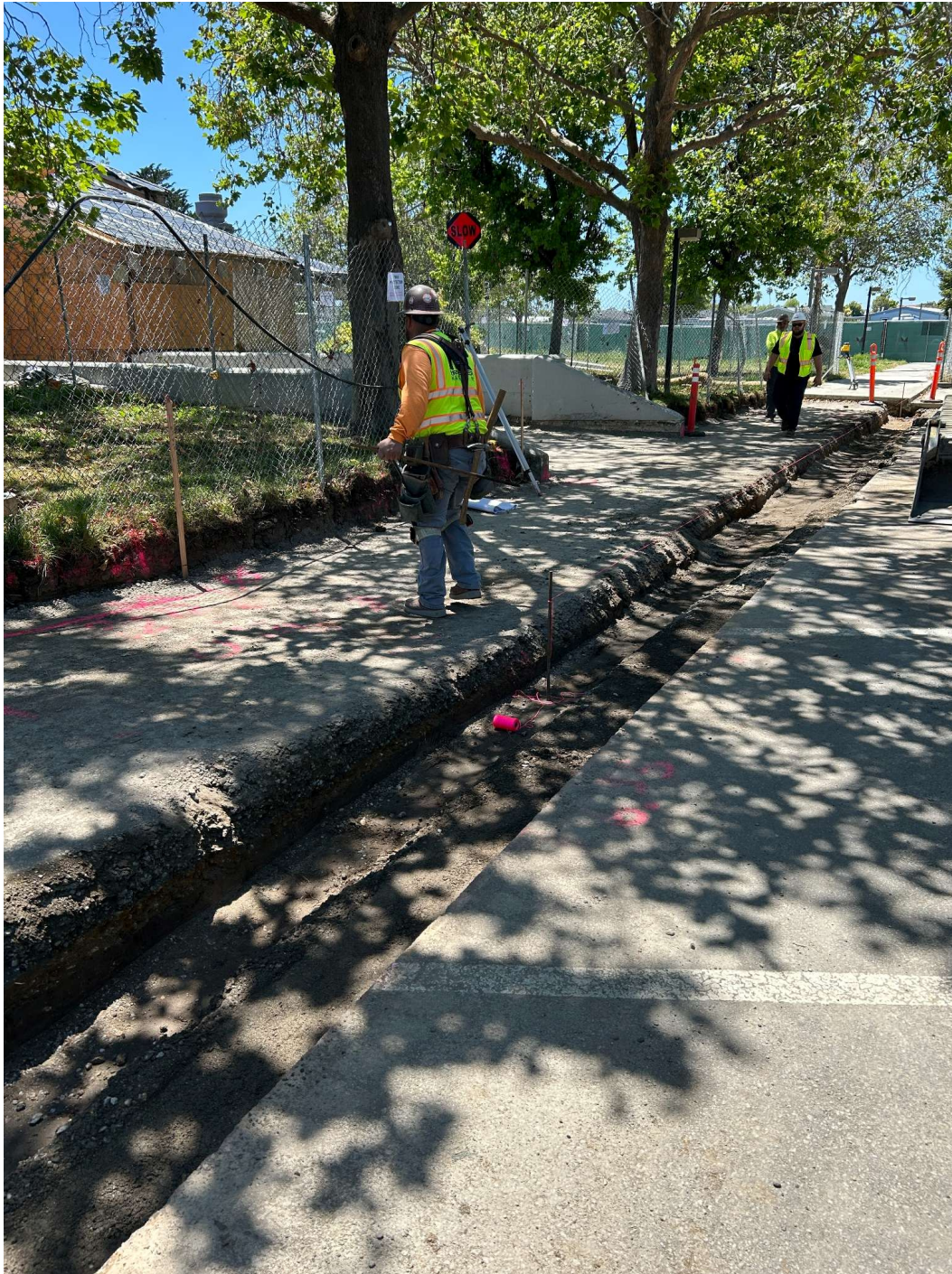
Crews trenching along sidewalk for underground utilities.
