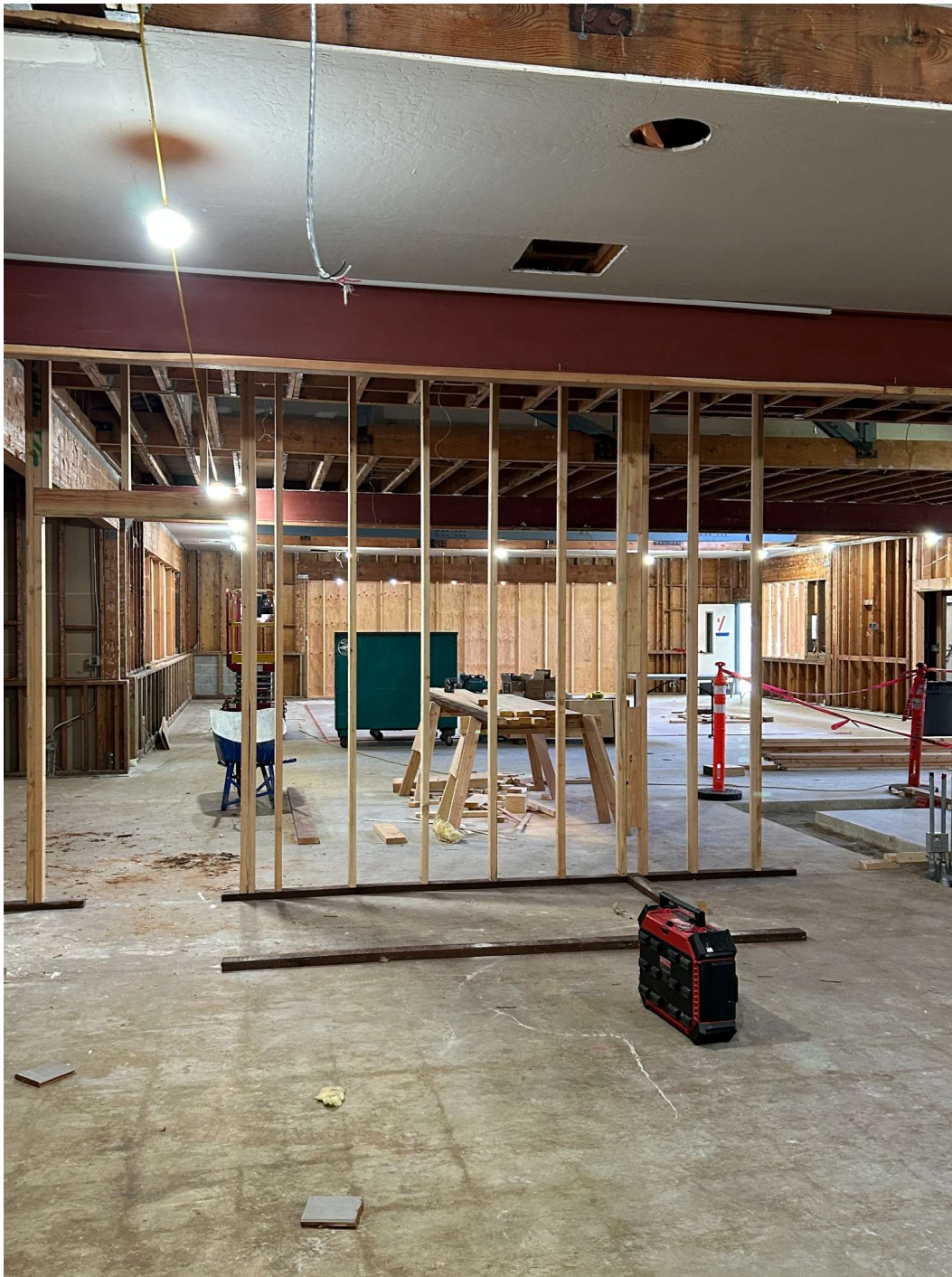
Interior stud framing walls in progress with open ceiling.
