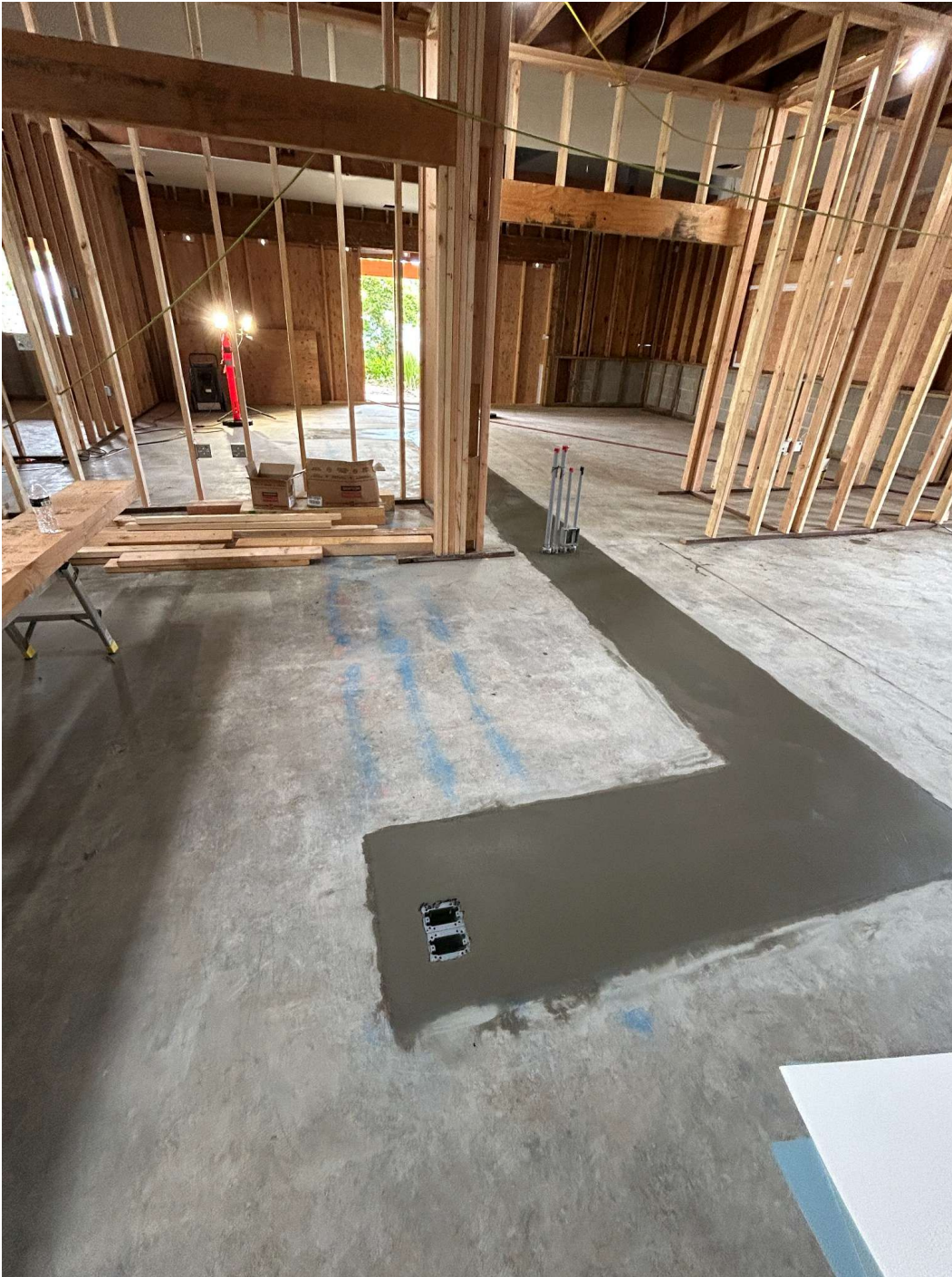
New concrete patch inside building covering utility trench.
