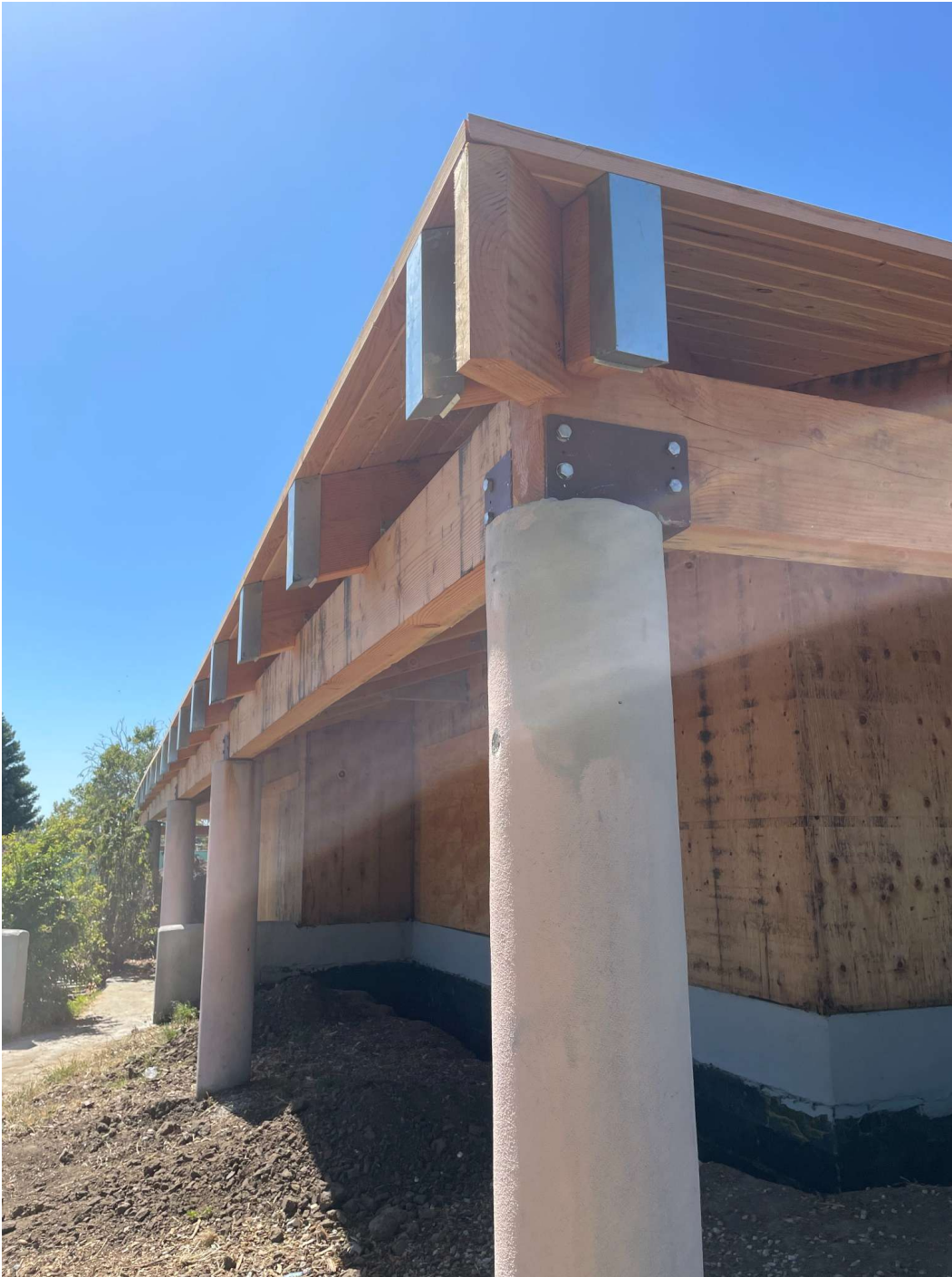
Close-up of new beams and steel brackets installed on concrete support columns.
