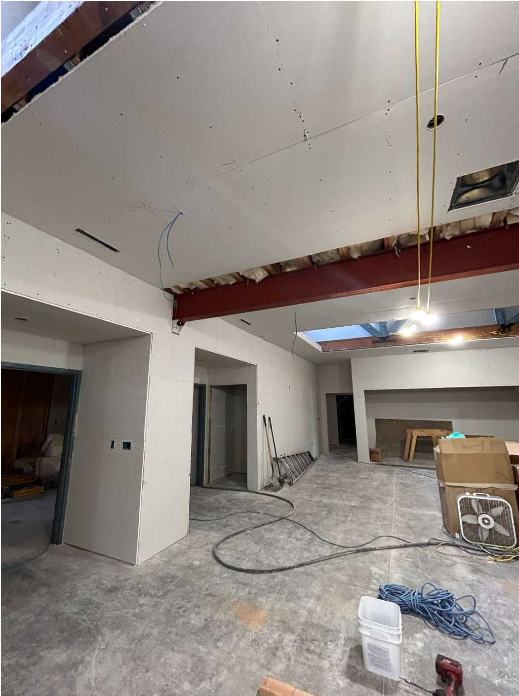
Interior drywall installed in large main room; steel beams and electrical rough-in visible.
