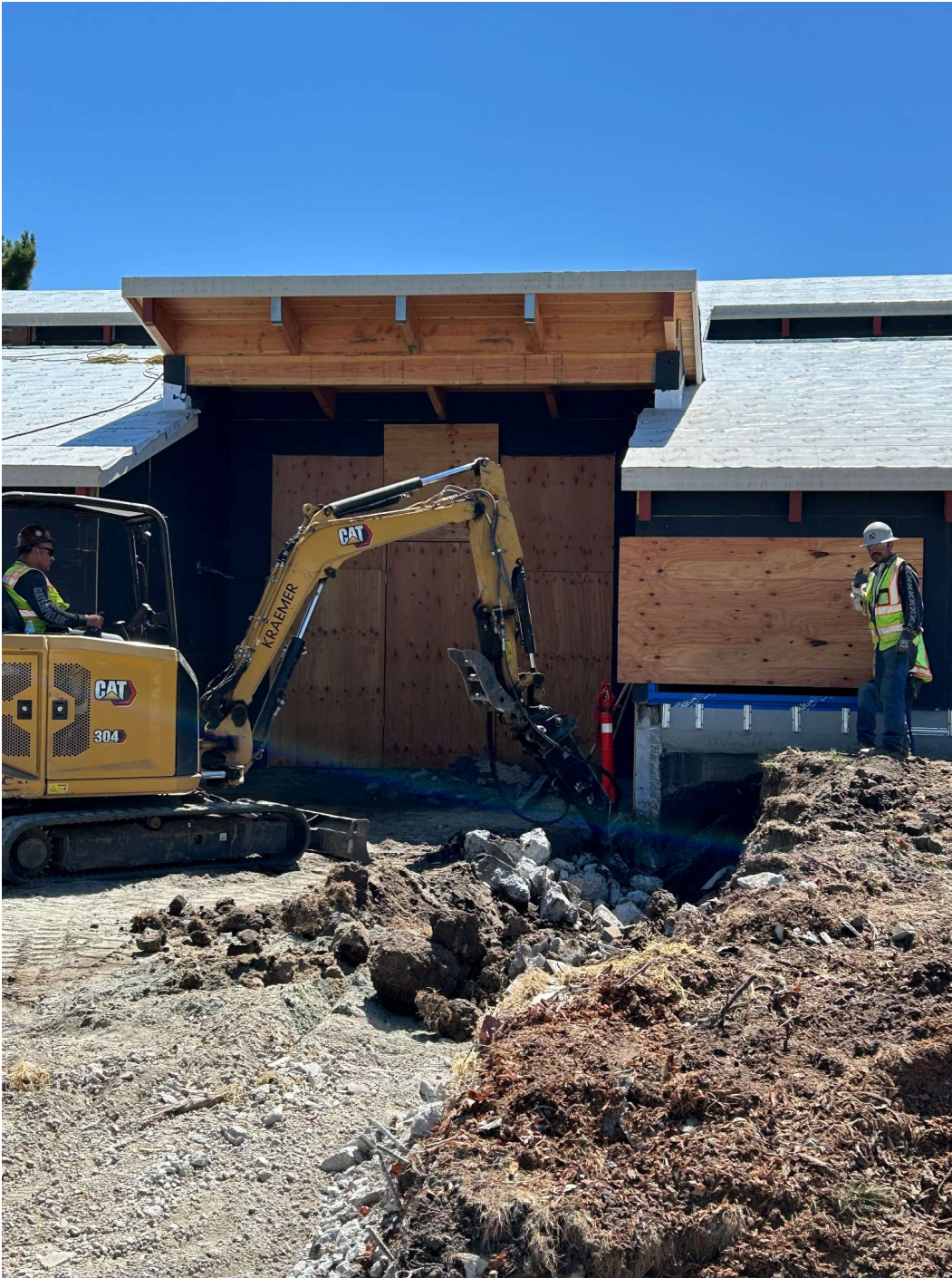
Excavation and demolition at the building entry; equipment breaking up existing concrete.
