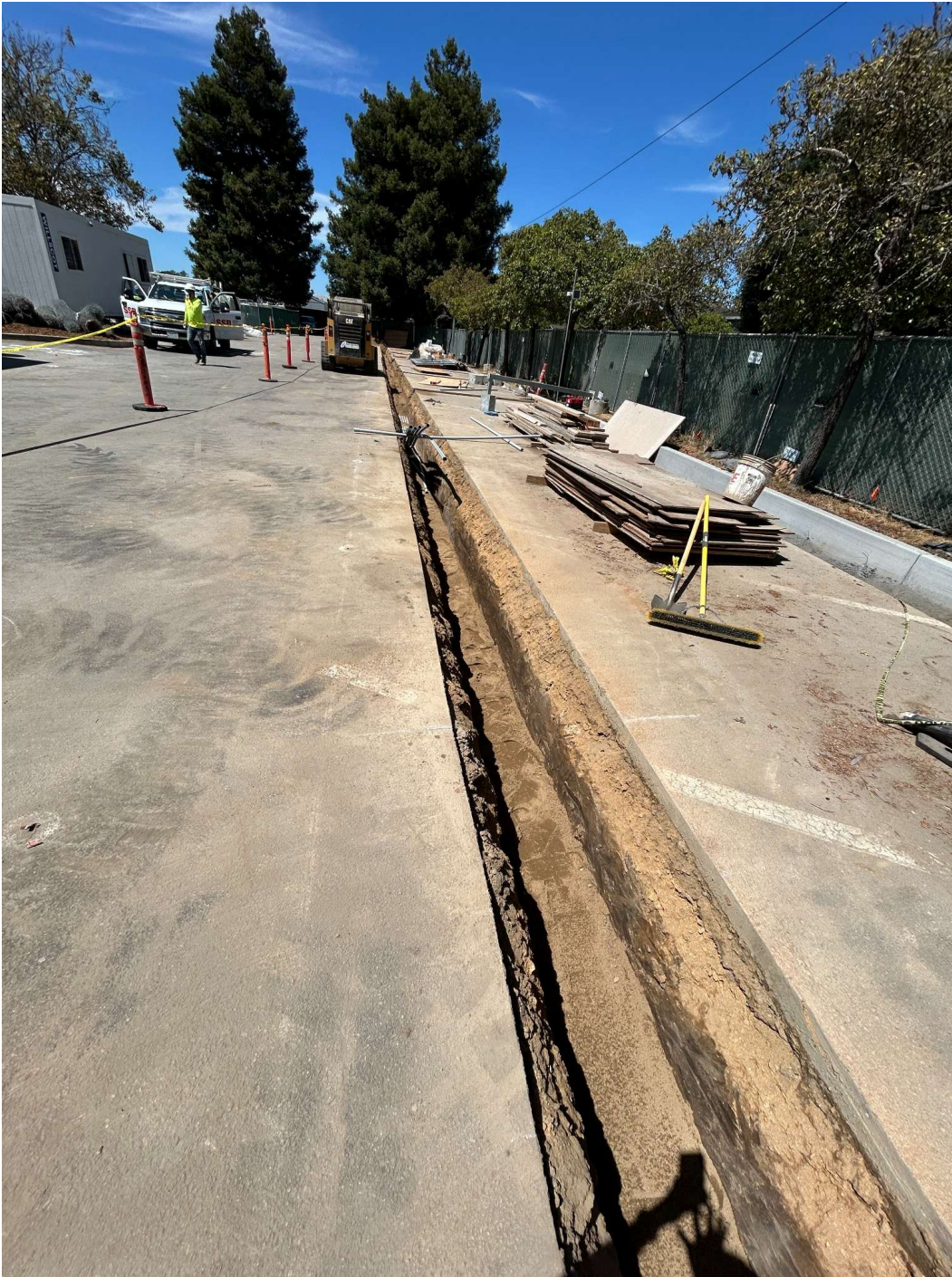
Long trench cut through asphalt for conduit installation, extending approximately 300 feet.
