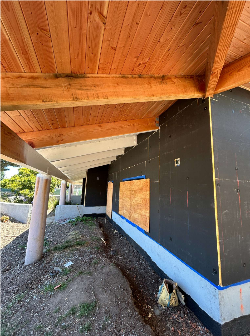
View of new waterproofing along the exterior wall, with wood ceiling soffit above.
