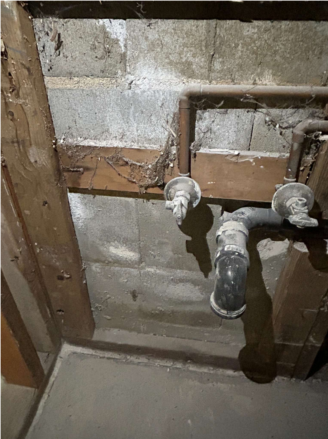
Exposed plumbing pipes at restroom wall during rough-in stage.
