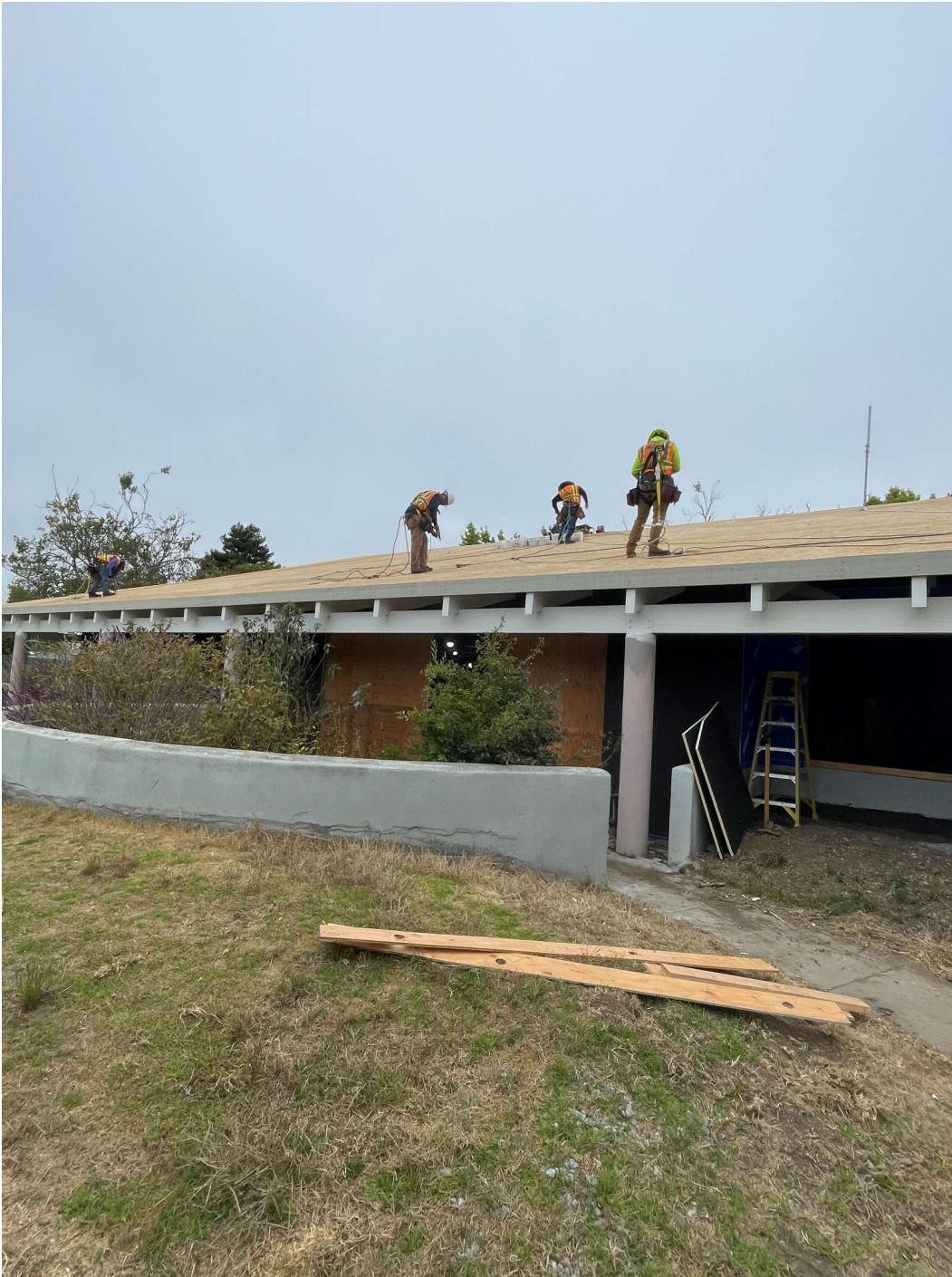
Multiple workers fastening new roof sheathing in place.
