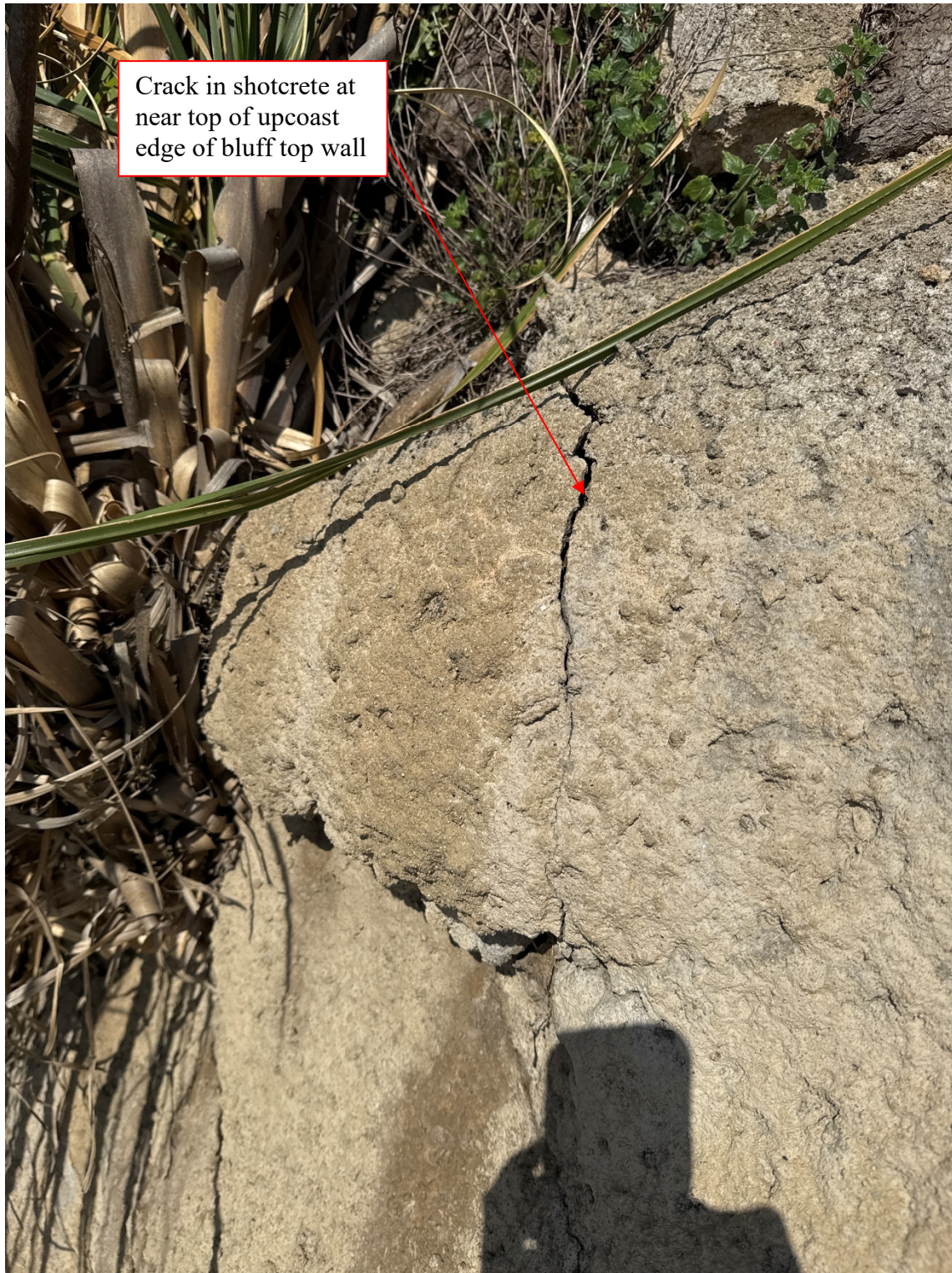
Photo 3: Crack in Shotcrete near top of upcoast end of bluff top retaining wall - 2 April 2025
