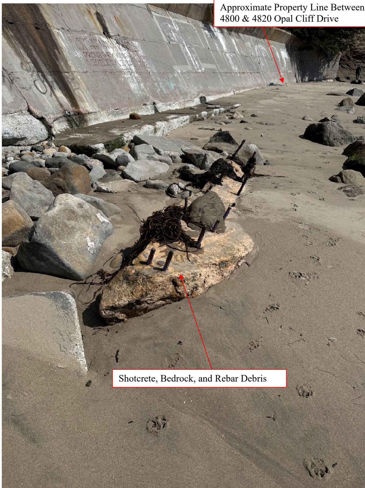
Photo 13: Downcoast View of Seawall - 2 April 2025
