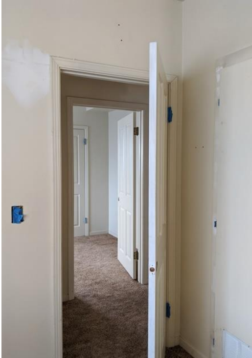
Interior of Central Wing of House. Viewed facing north. January 2020. (Photo by Leslie Dill)
