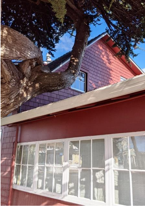
South Elevation. Showing upstairs windows and enclosed former front porch. Viewed facing northeast. January 2020. (Photo by Leslie Dill)
