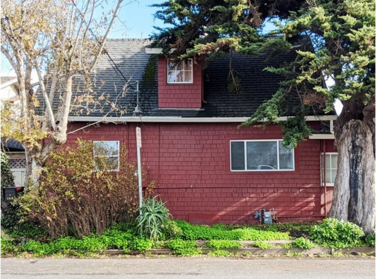
North Half of Front of House. Viewed facing east. January 2020. (Photo by Leslie Dill)
