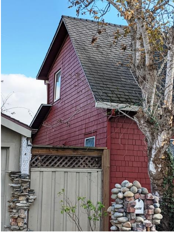
North Elevation. Viewed facing southeast. January 2020. (Photo by Leslie Dill)
