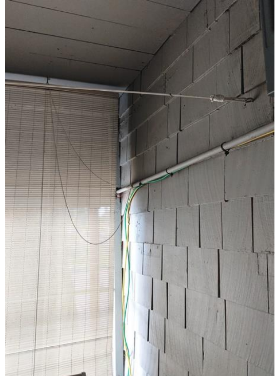
Interior of Enclosed Former Front Porch. Viewed facing northwest. January 2020. (Photo by Leslie Dill)
