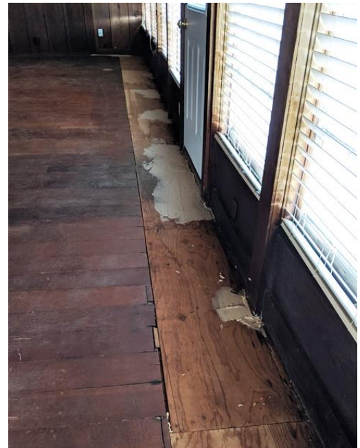
Detail of Living Room Floor Repair. Viewed facing north. January 2020. (Photo by Leslie Dill)
