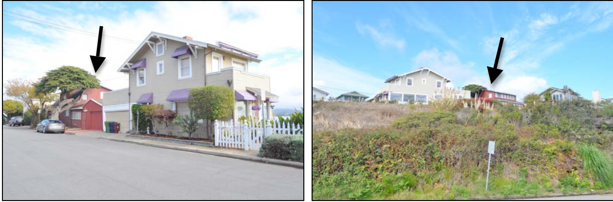
Figures 5 and 6. Left image shows the rhythm of gable roofs and false front roofs along Prospect Avenue, looking north, with the subject property indicated by an arrow. Right image views the variety of historic rooflines along the ridge looking northwest from Cliff Drive.
