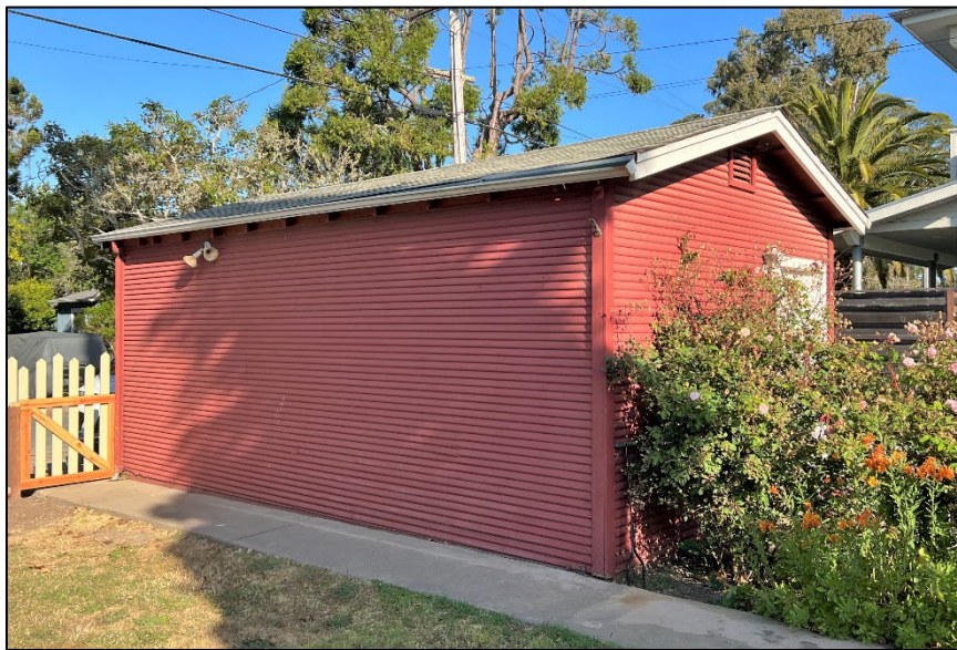
Photograph 8: Garage viewed from the east corner, showing lack of fenestration and ornamentation on the southeast side. Camera facing west, June 22, 2022.
