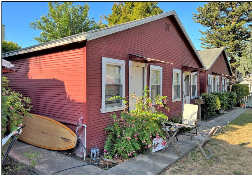
Photograph 3: Unit B (left) and Unit A (right) at 204 Hollister Avenue. Camera facing south, June 22, 2022.
