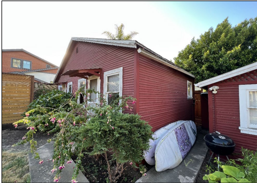
Photograph 4: Unit C, located at 204 Hollister Avenue. Camera facing east, June 22, 2022.
