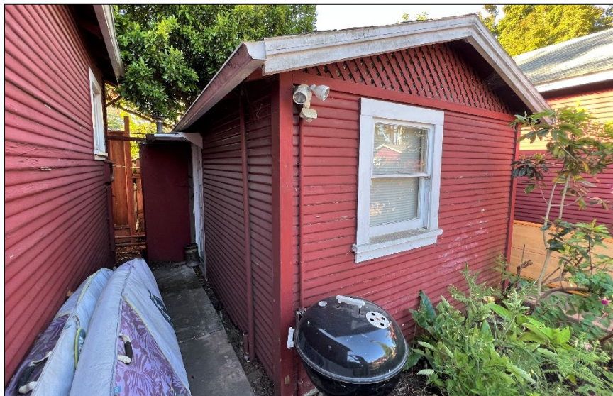
Photograph 10: Storage building viewed from the north corner, showing fenestration on the northwest gable end and the secondary entrance on the northeast side. Camera facing south, June 22, 2022.
