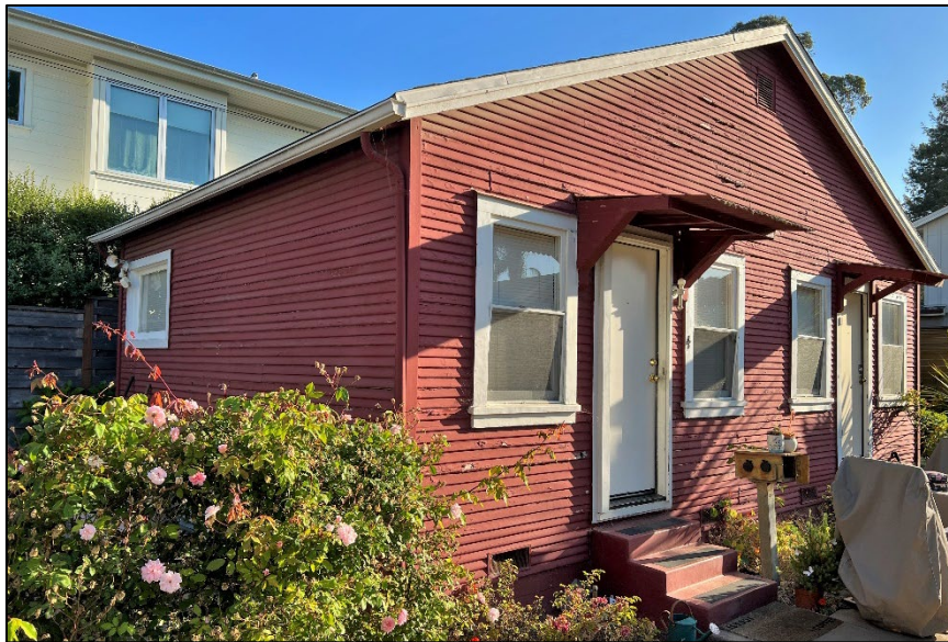
Photograph 5: Unit D, located at 206 Hollister Avenue. Camera facing north, June 22, 2022.
