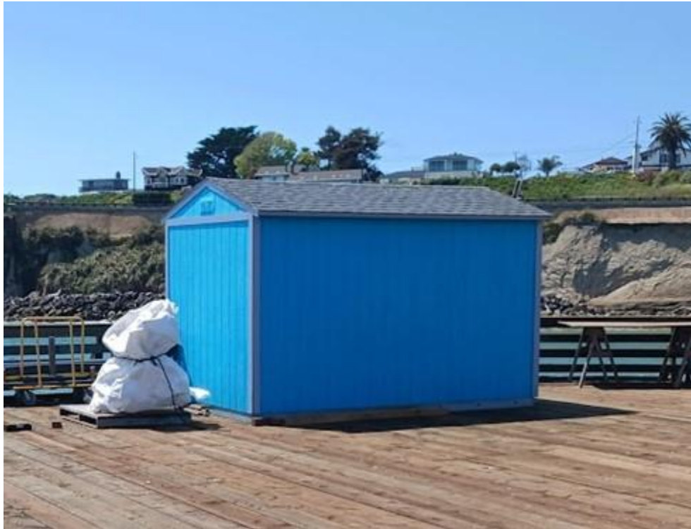
Figure 4. Existing Storage Shed (above)
