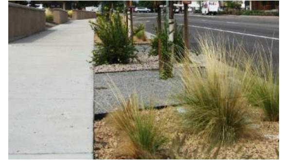
STABILIZED GRAVEL AREA AROUND TREE WELL
