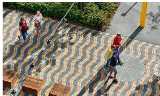
SPECIAL PAVING EXAMPLE - CURVED UNIT PAVERS
