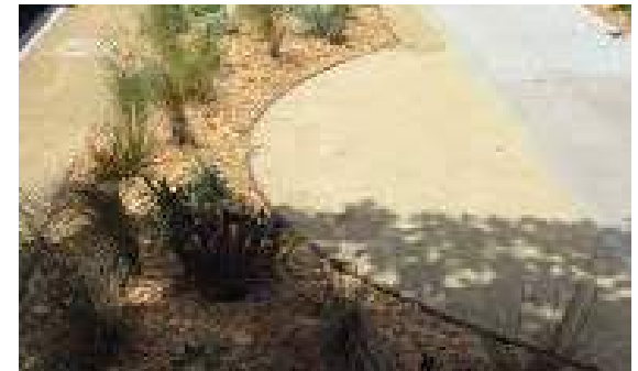
DG SHOULDER ALONG SIDEWALK
