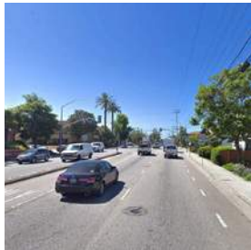
41ST AVENUE AT BROMMER STREET
