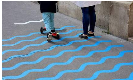
SPECIAL PAVING EXAMPLE - THERMOPLASTIC APPLICATION
