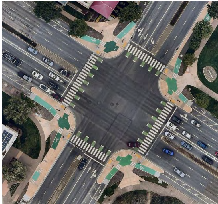
Example protected intersection features for bikes and peds at a signalized intersection (Fremont)
