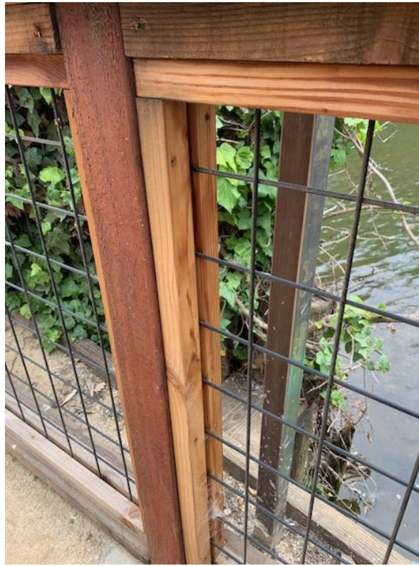
Hog Wire framed in wood railing along Riverview Path
